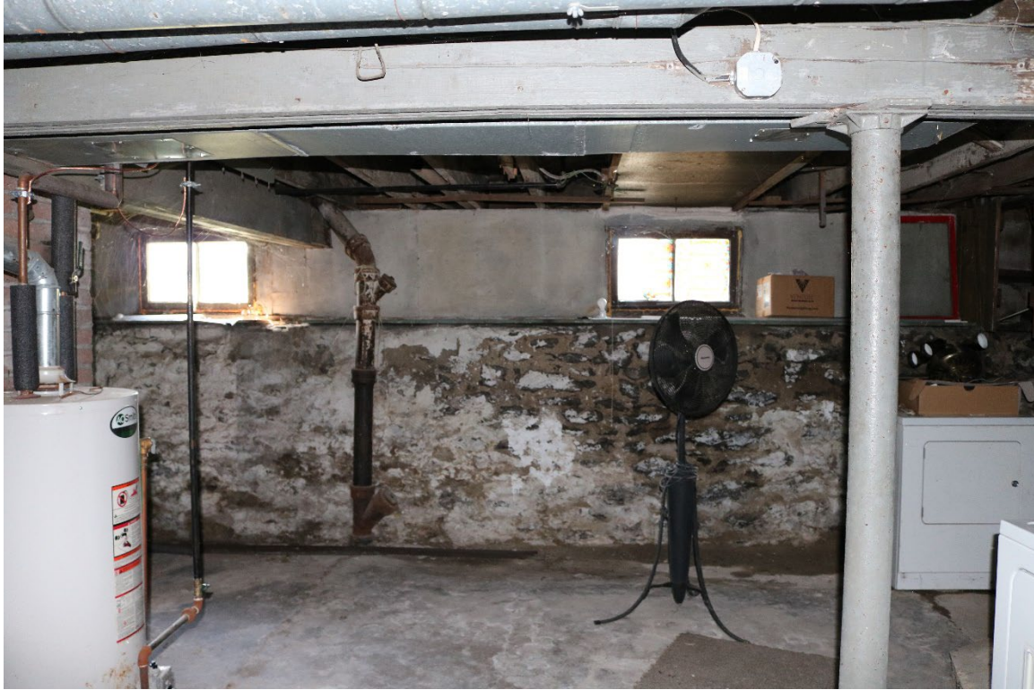
44. View of basement, facing north ( Commonwealth 2022 ).
