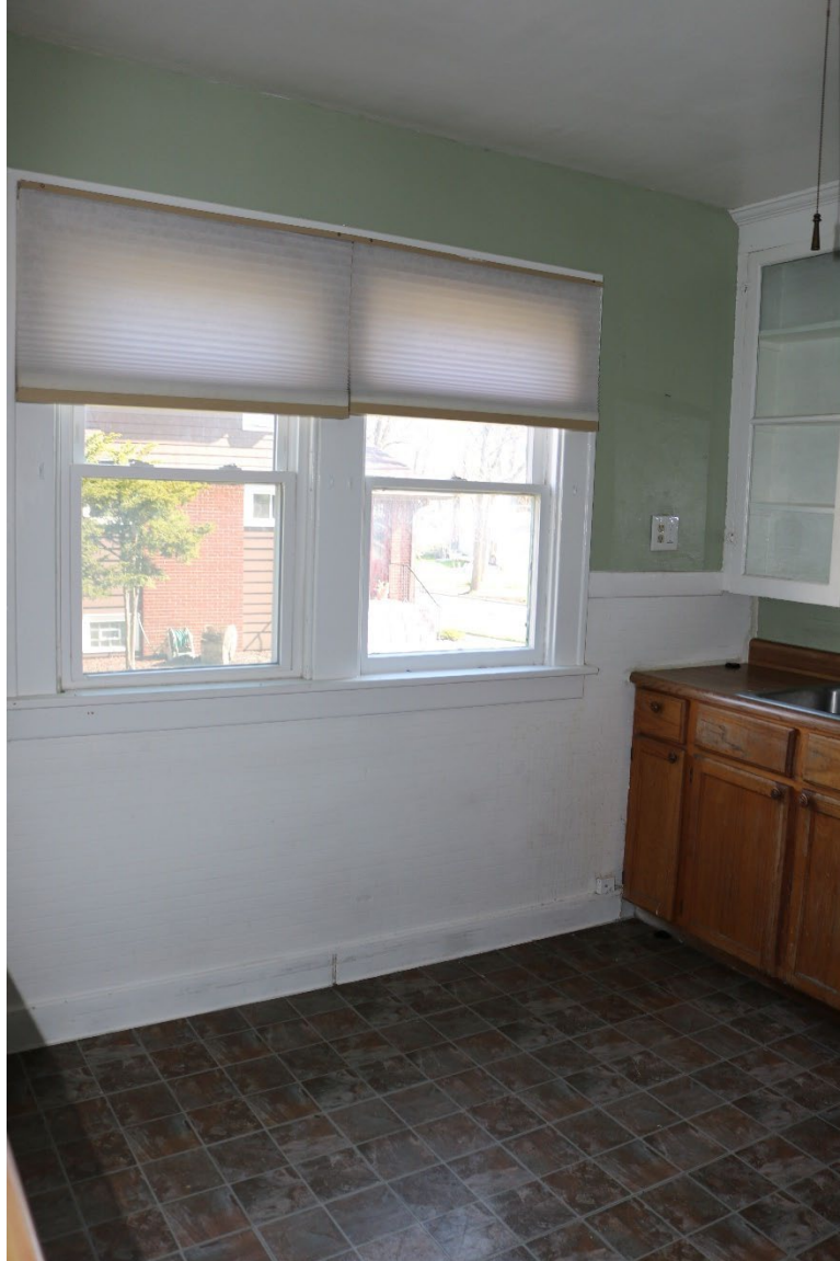
26. View of west wall in kitchen, facing northeast ( Commonwealth 2022 ).
