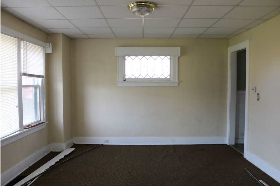
22. View of dining room, facing west ( Commonwealth 2022 ).
