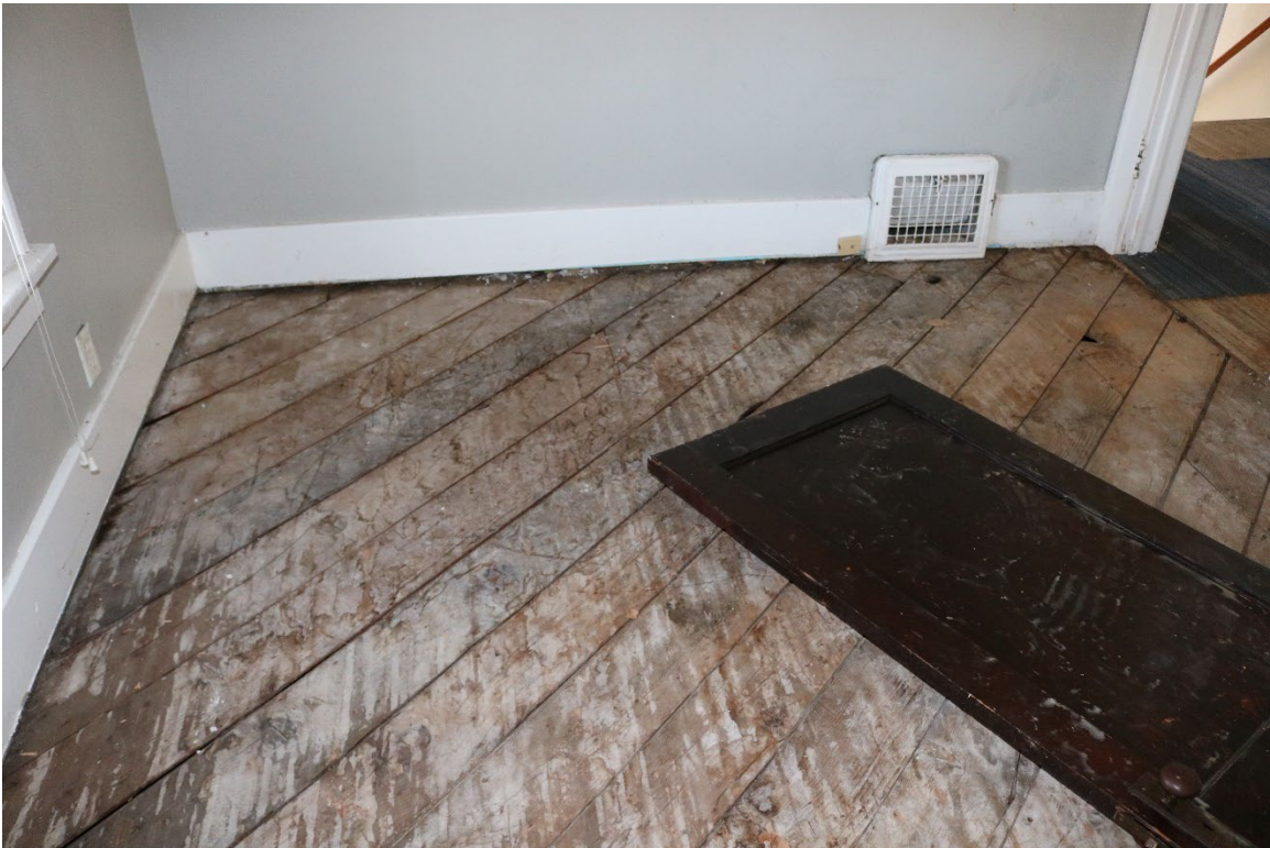
38. Detail of wood floor in southwest bedroom on second floor ( Commonwealth 2022 ).
