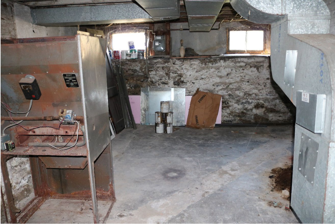
42. View of basement, facing south ( Commonwealth 2022 ).
