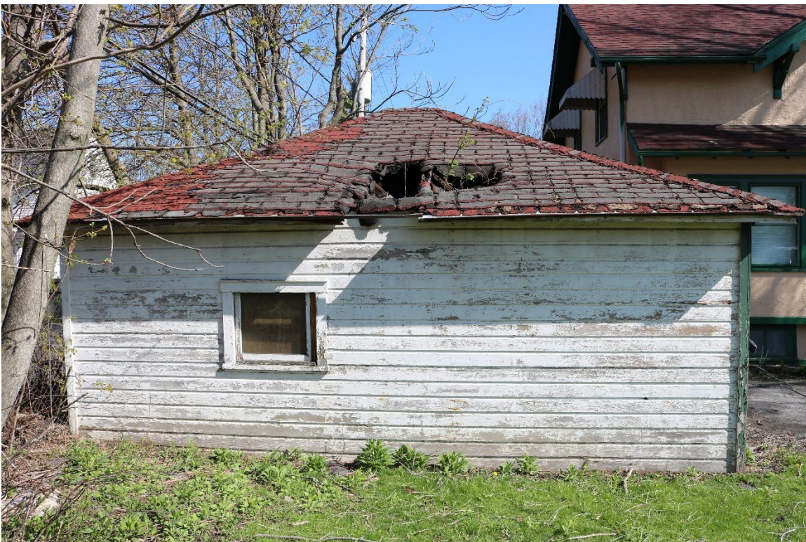
14. Direct view of south elevation of garage, facing west ( Commonwealth 2022 ).
