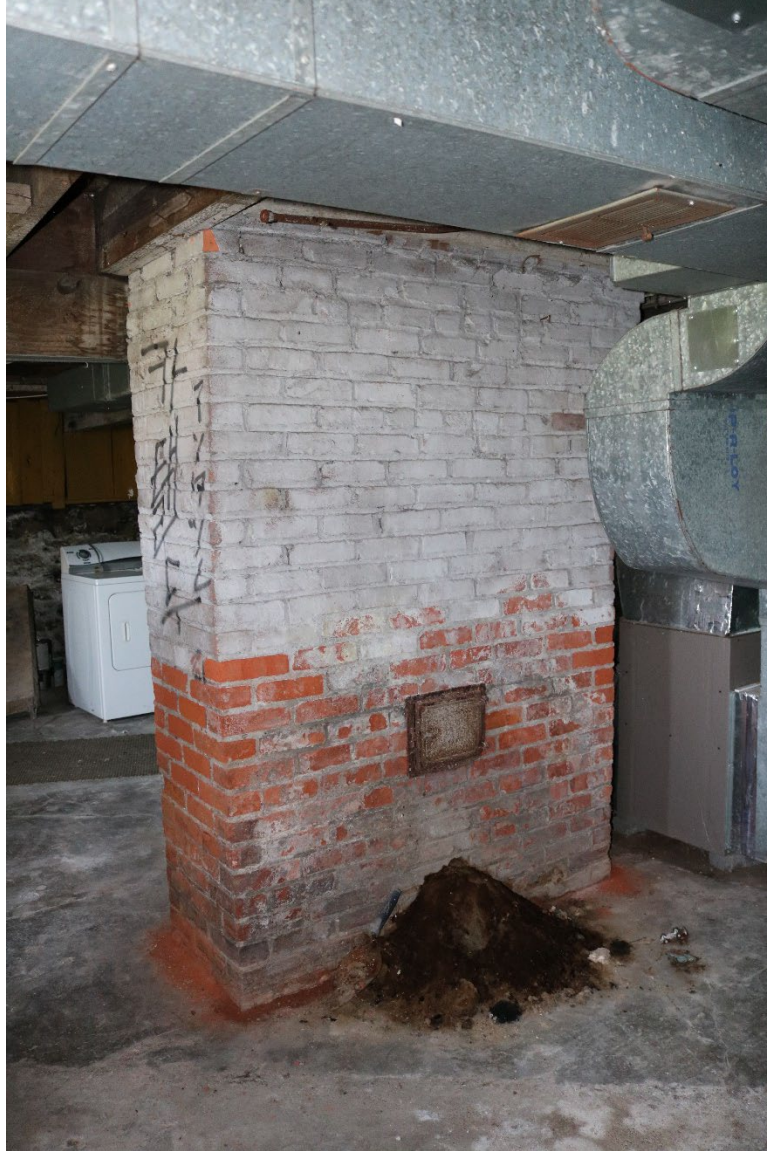
45. View of basement, facing west-northwest ( Commonwealth 2022 ).
