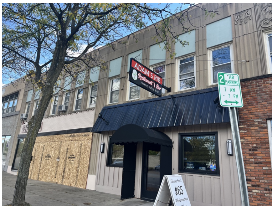
Figure 17. Primary (north) Façade, Hallie Wright
