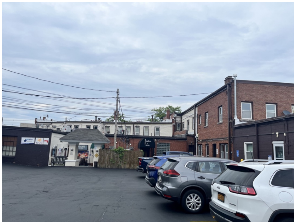
Figure 11. Rear Building, Facing South, Hallie Wright
