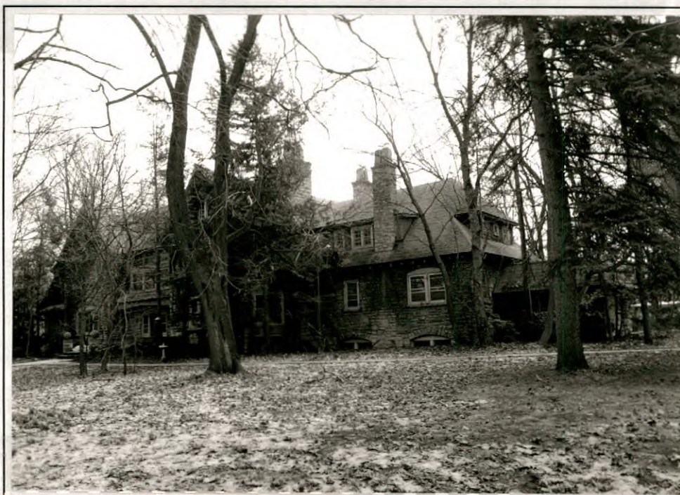
North and west elevations.
