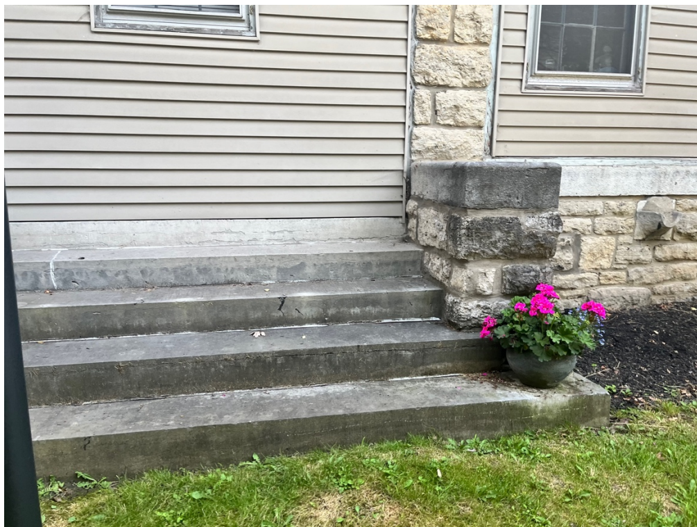
Figure 3. Southeast Elevation, Including Steps and Vinyl Siding
