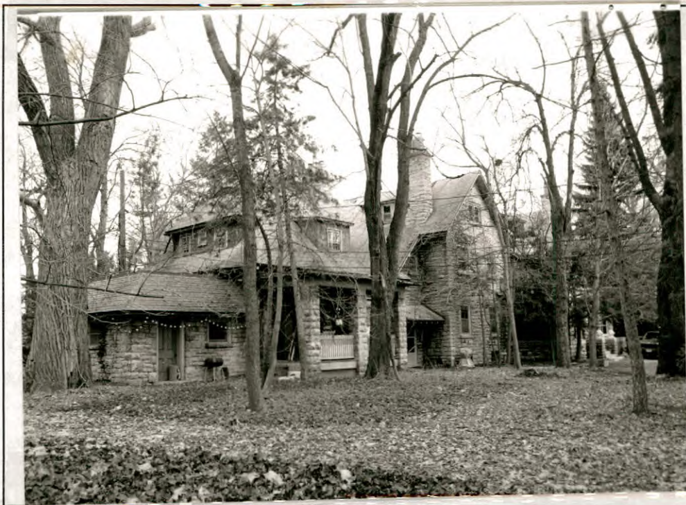
50 Getzville Road. West and south elevations.
