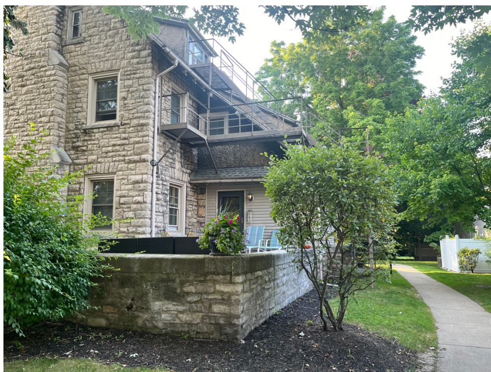
Figure 2. Southeast Elevation, Including Porch
