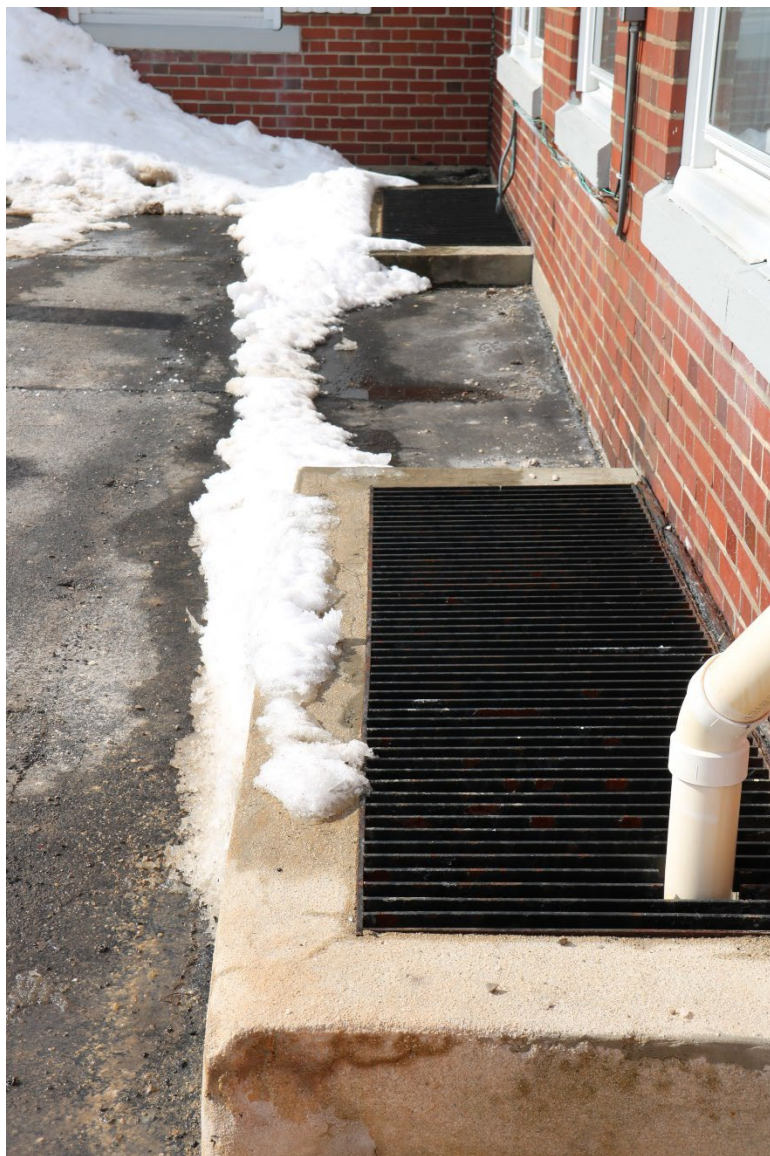
Photograph 24. Detail of basement window well along south façade, 4467 Main Street, facing west.
