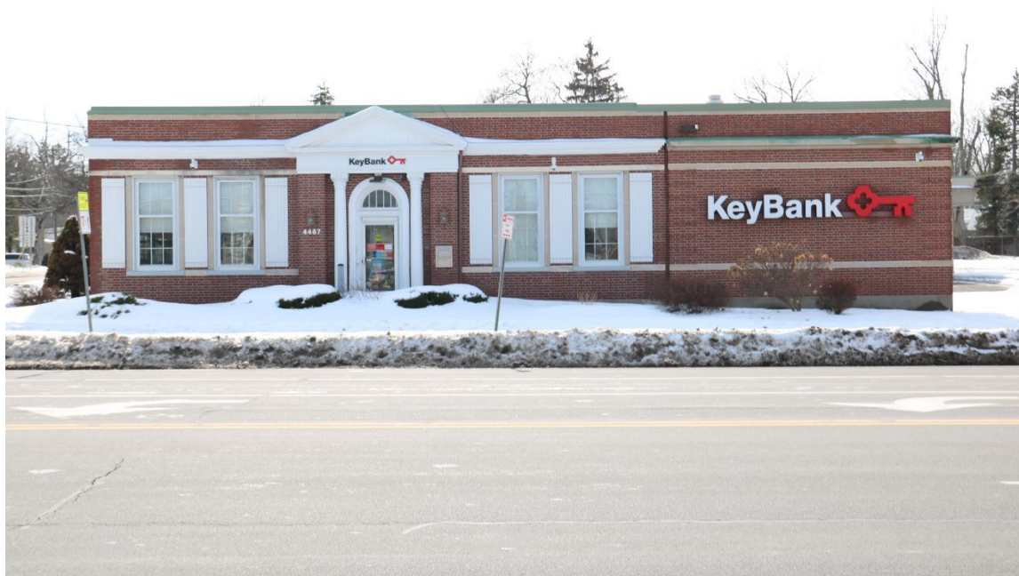
Photograph 5. South façade, 4467 Main Street, facing south.
