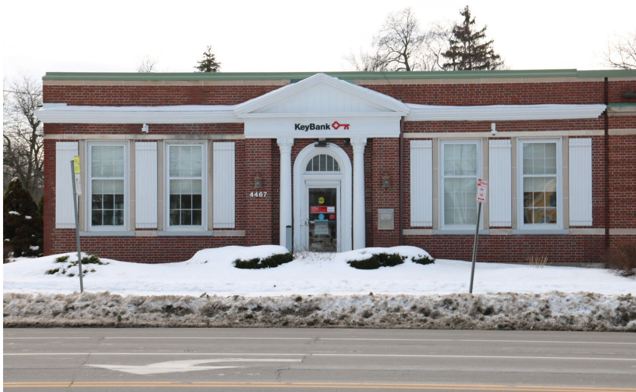
Photograph 6. Detail of south façade, 4467 Main Street, facing south.
