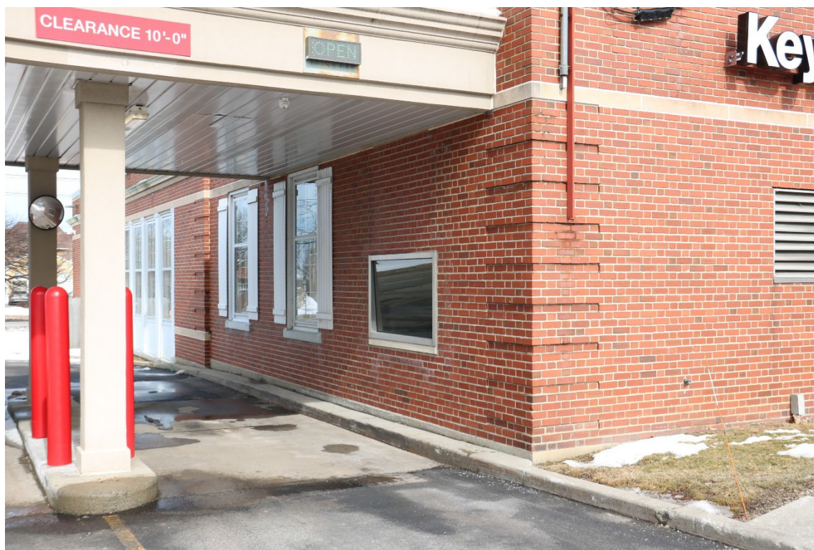
Photograph 16. Drive-through lane with bank teller window, 4467 Main Street, facing northeast.
