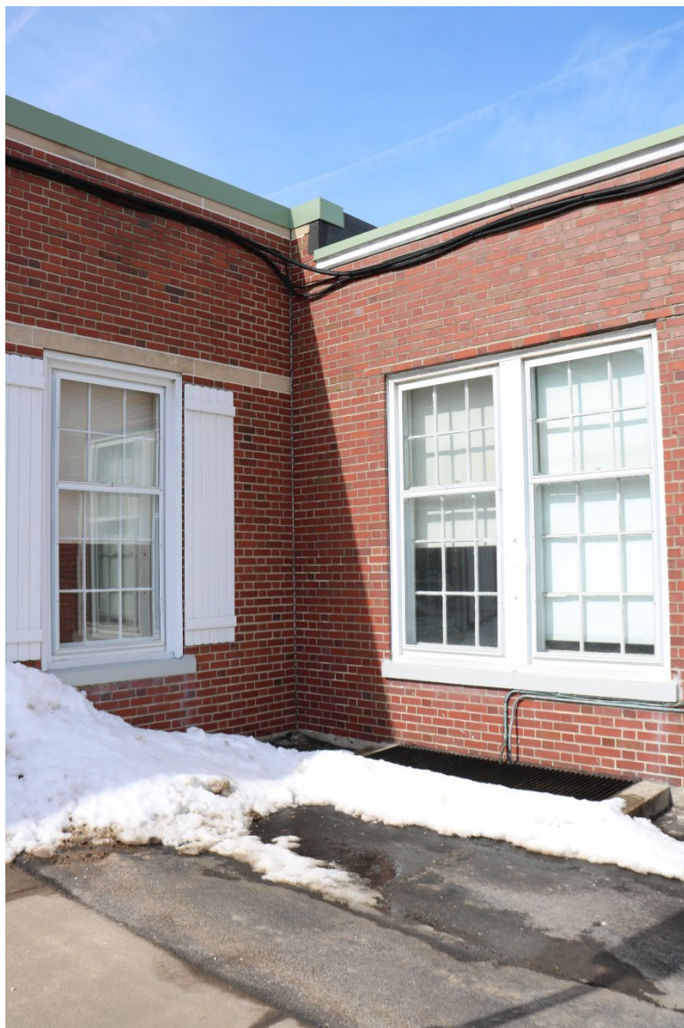
Photograph 25. Detail of addition and main block, 4467 Main Street, facing northwest.
