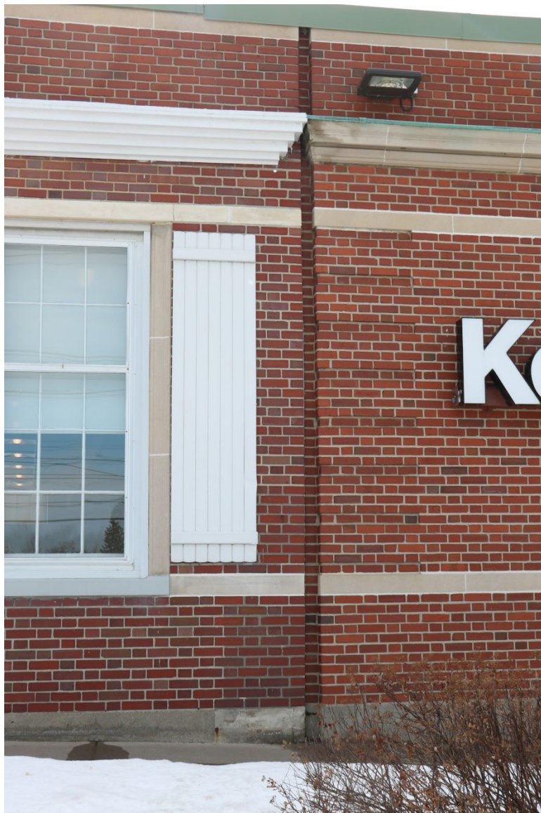
Photograph 20. Detail of north facade, 4467 Main Street, facing south.
