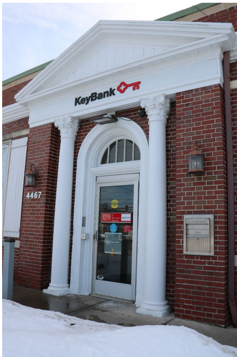
Photograph 19. Detail of north entrance, 4467 Main Street, facing southeast.
