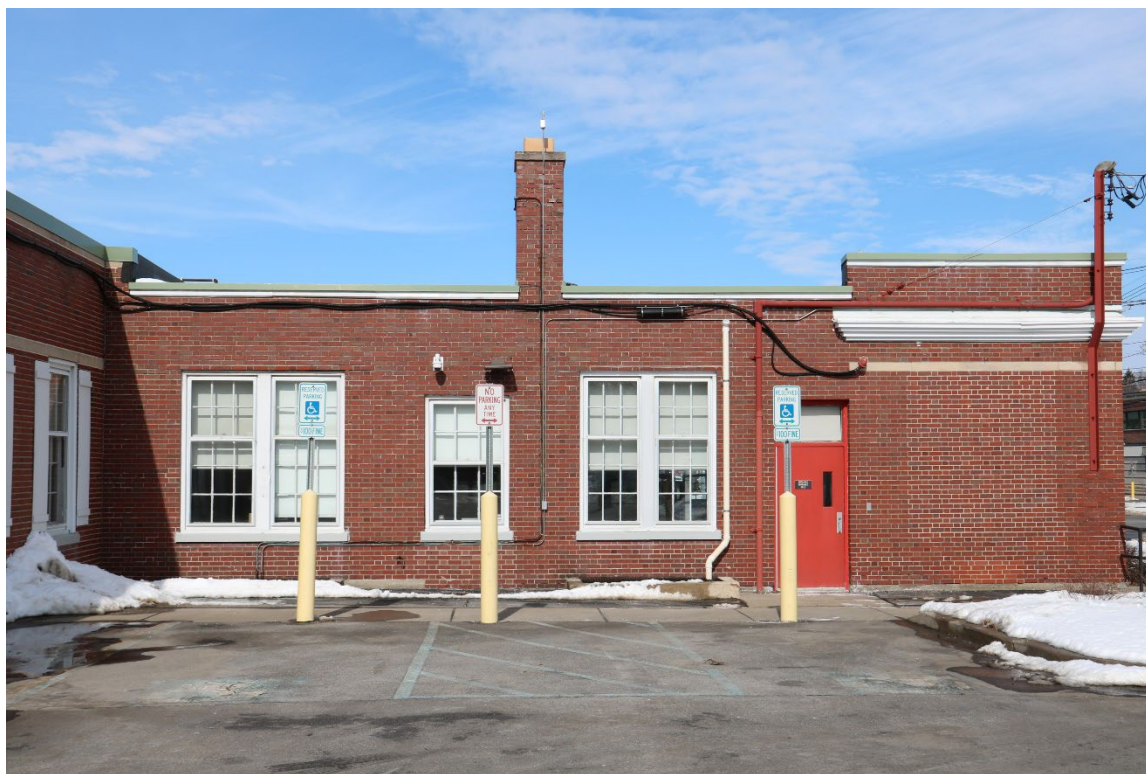
Photograph 11. Detail of south façade, 4467 Main Street, facing north.
