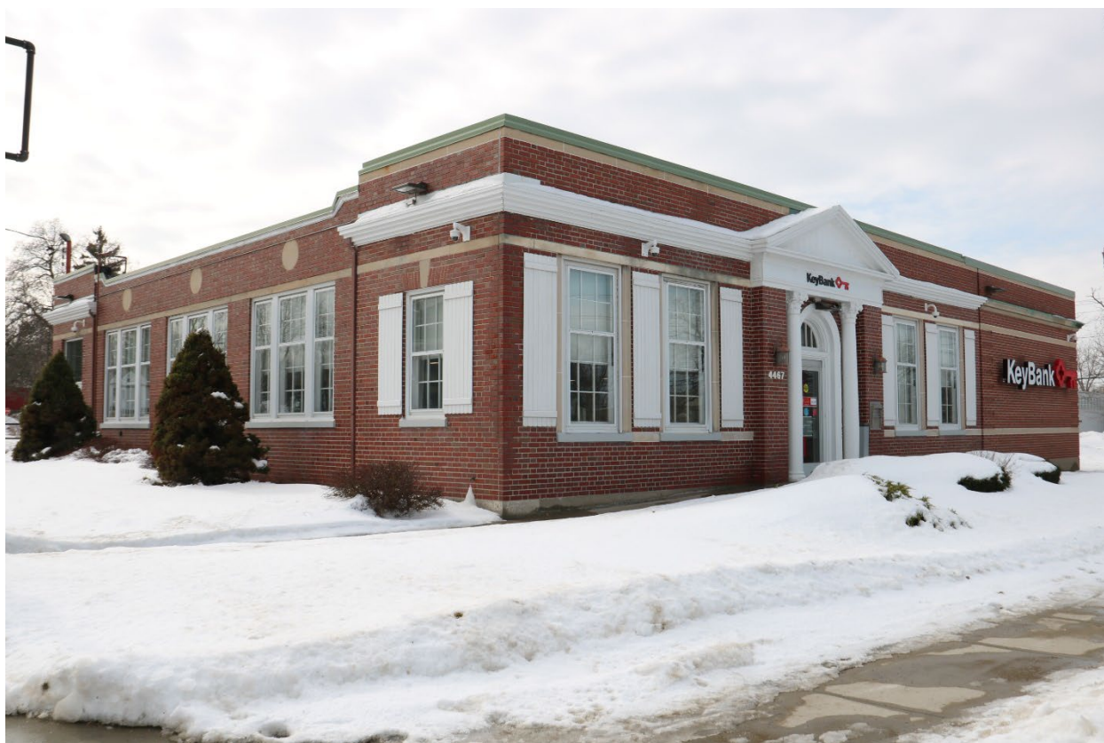
Photograph 7. East and north facades, 4467 Main Street, facing southwest.
