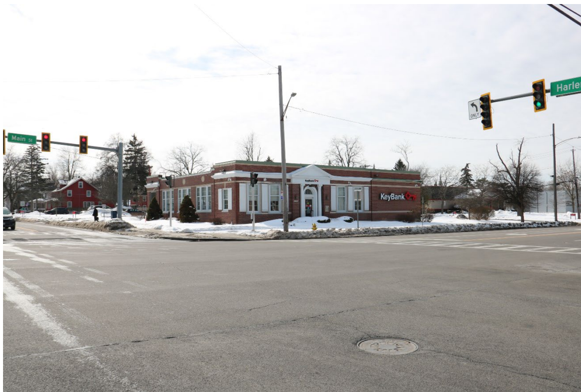
Photograph 1. Setting view of 4467 Main Street, facing southwest.
