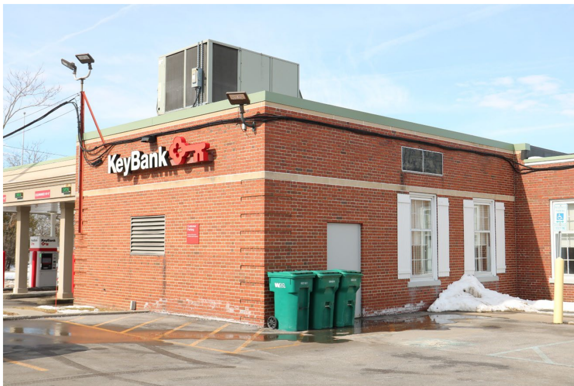
Photograph 13. South and east façades of addition, 4467 Main Street, facing west.
