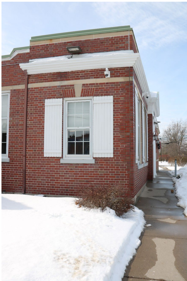
Photograph 21. Detail of east window opening and cornice, 4467 Main Street, facing west.
