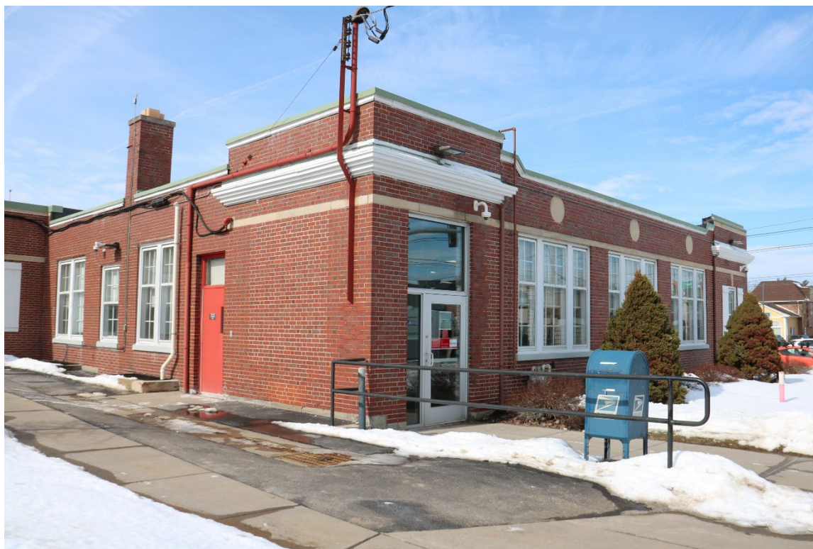
Photograph 10. South and east facades, 4467 Main Street, facing northwest.
