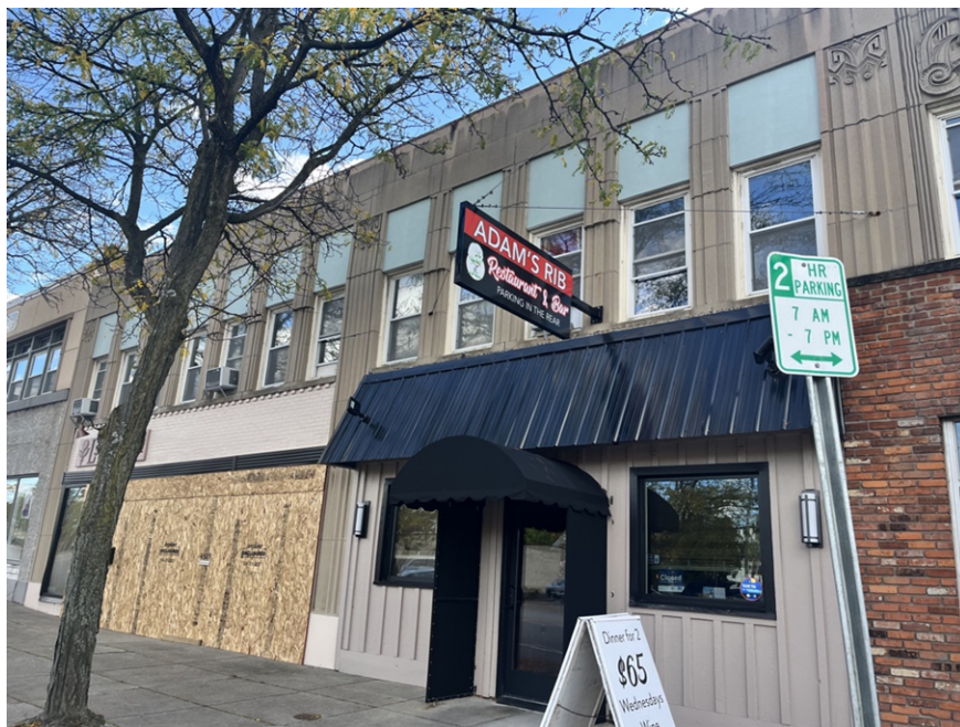
Figure 17. Primary (north) Façade, Hallie Wright
