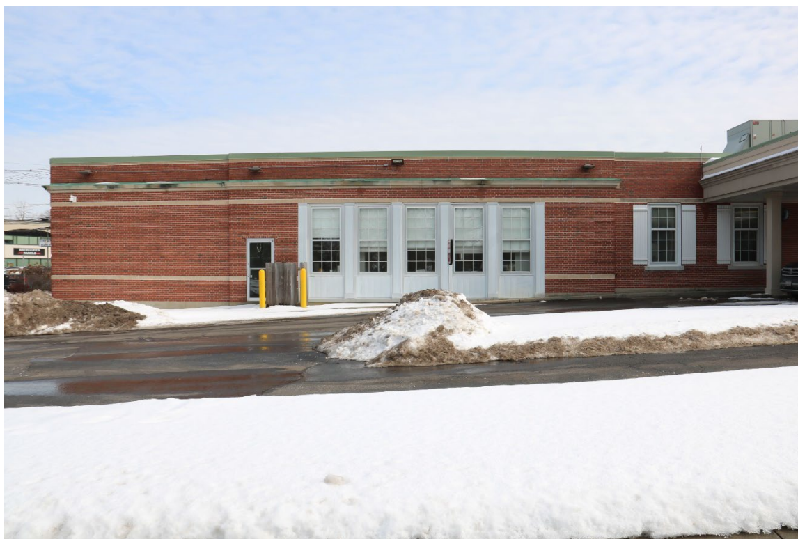
Photograph 15. Drive-through canopy addition west façade, 4467 Main Street, facing west.
