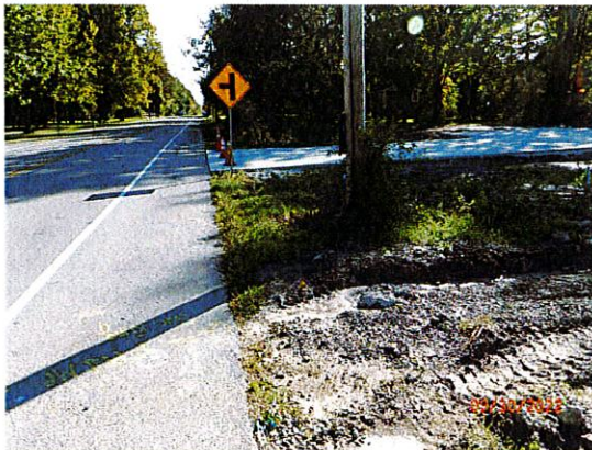
Picture from field inspection by Planning Staff on September 30, 2022; 695 Casey Road looking east at the potential location of a sidewalk.
