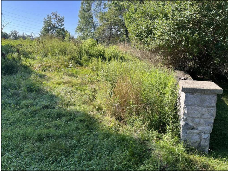
Photograph 3. APE from the northwest corner, looking south.
