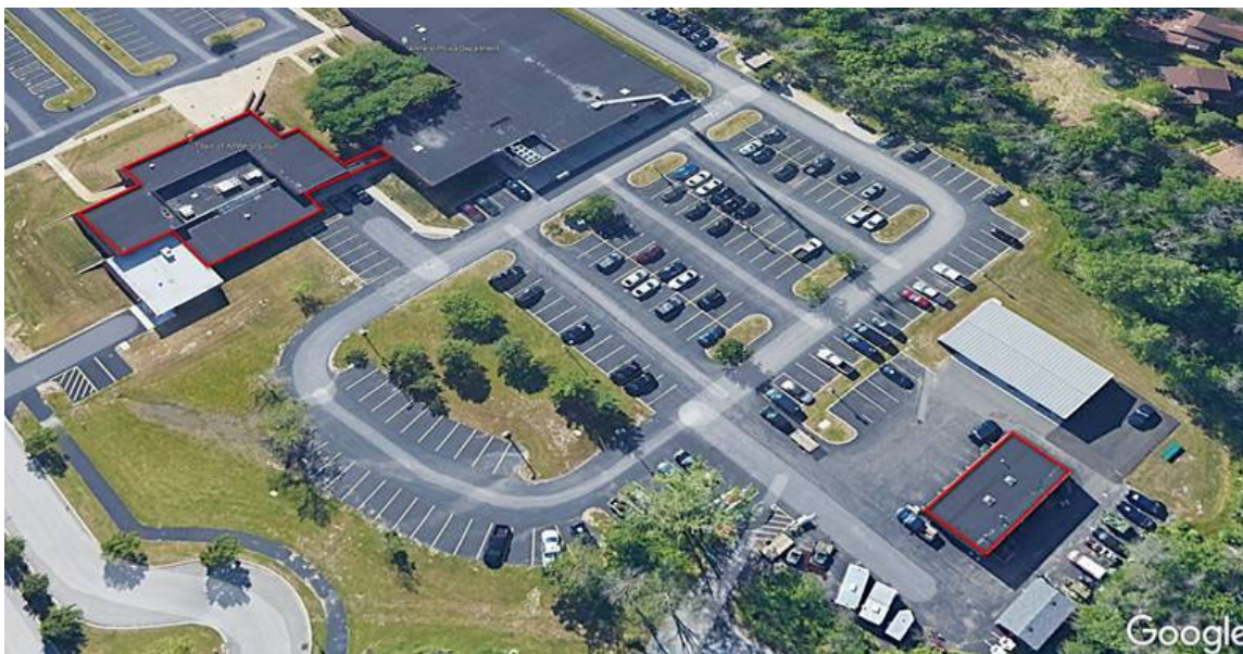
Town Court Building (left) and Police Maintenance Garage (right) with highlighted roof areas
