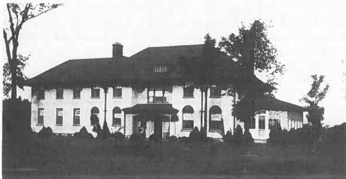
ESTATE OF FRANK L. BAPST, EGGERTSVILLE ROAD
