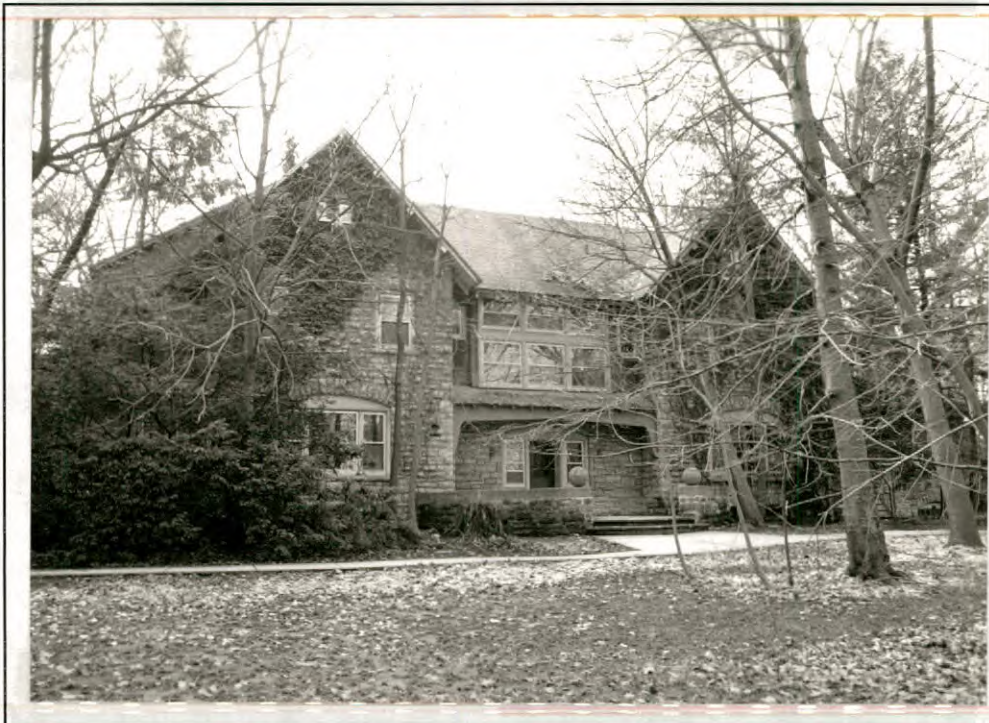
50 Getzville Road. North elevation.
