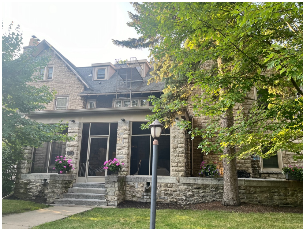
Figure 1. Primary (South) Façade
