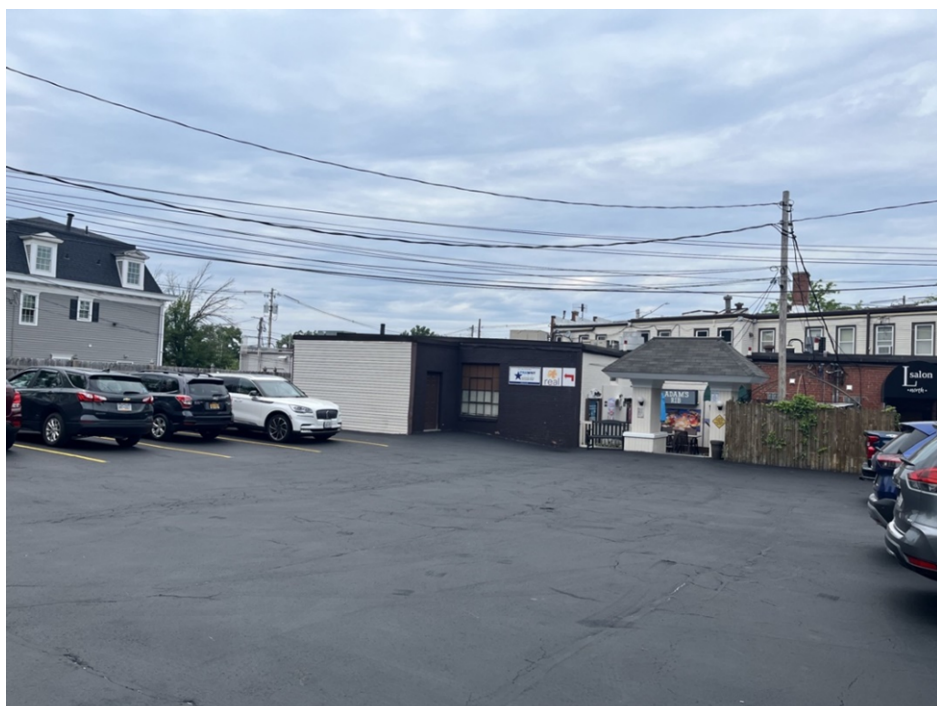
Figure 12. Rear Building, Facing Northwest, Hallie Wright
