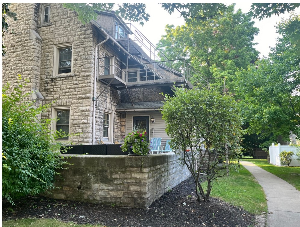
Figure 2. Southeast Elevation, Including Porch
