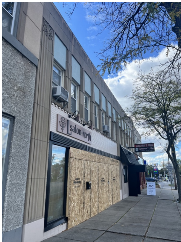
Figure 13. Primary (northeast) Façade, Hallie Wright
