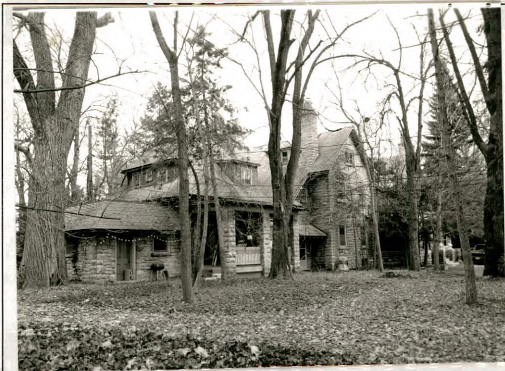
50 Getzville Road. West and south elevations.
