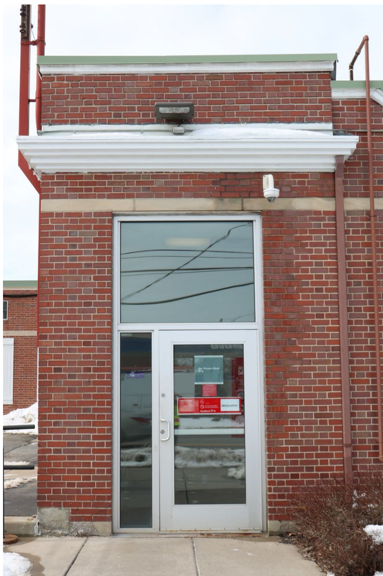
Photograph 23. Detail of east entrance, 4467 Main Street, facing west.
