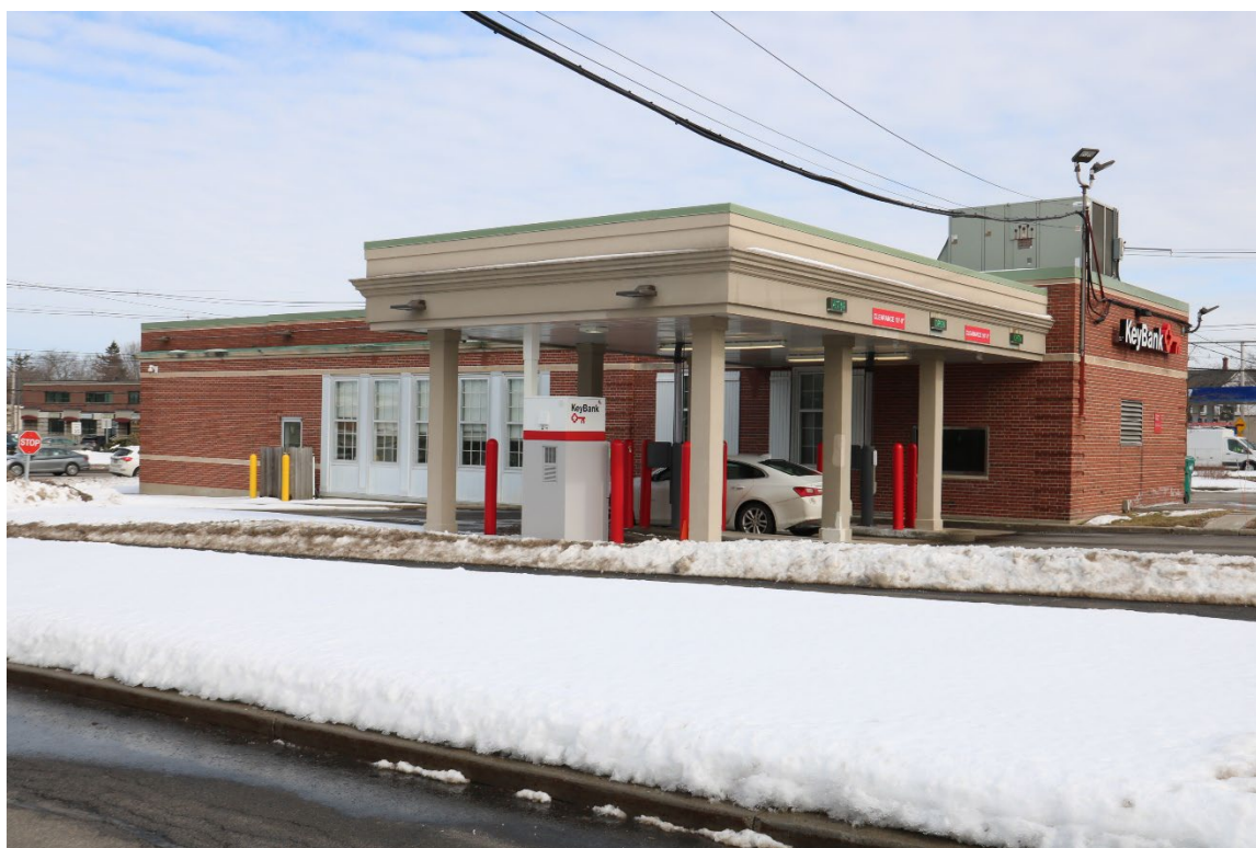
Photograph 14. Drive-through canopy addition west façade, 4467 Main Street, facing northeast.
