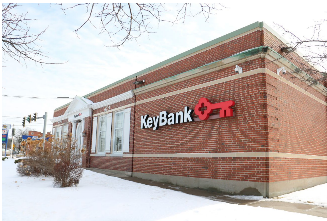
Photograph 16. West façade, 4467 Main Street, facing east-southeast.
