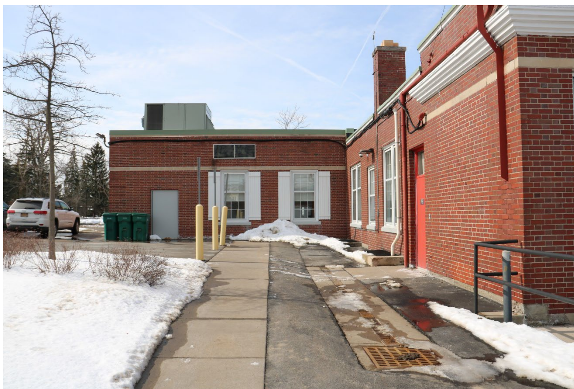
Photograph 12. East façade of addition and south façade of main block, 4467 Main Street, facing west.
