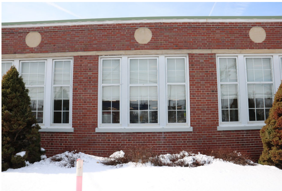
Photograph 22. Detail of east façade, 4447 Main Street, facing west.
