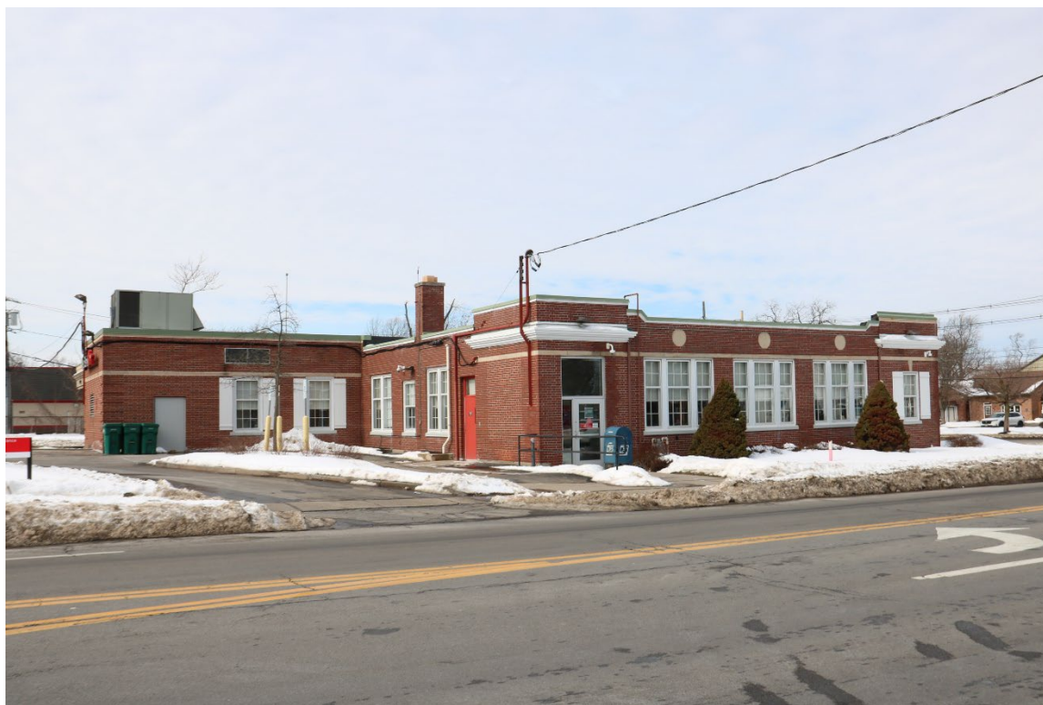
Photograph 9. Oblique view of 4467 Main Street, facing west-northwest.
