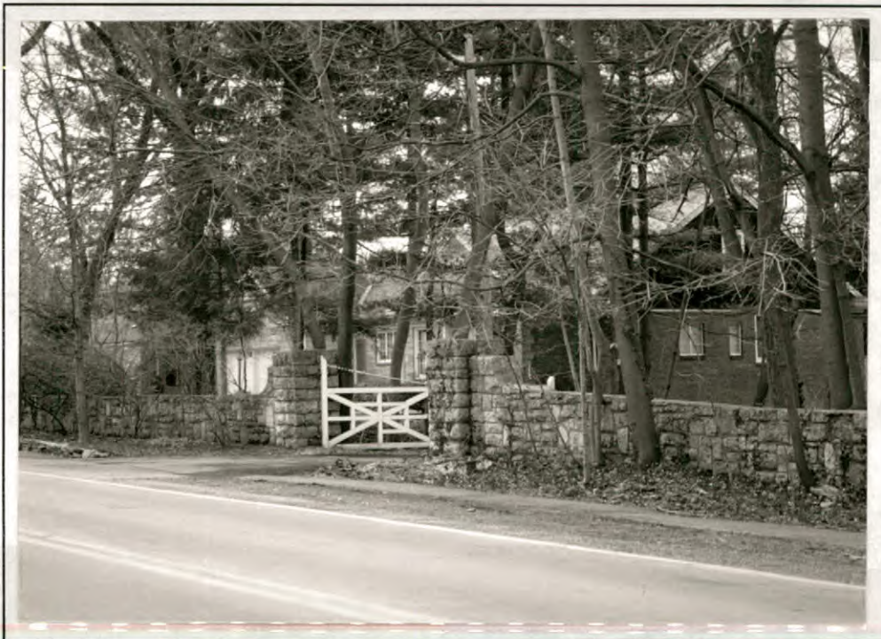
Stone wall at entrance on Getzville Road.
