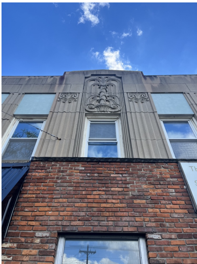
Figure 17. Primary (north) Façade, Frozen Fountain Detail, Hallie Wright
