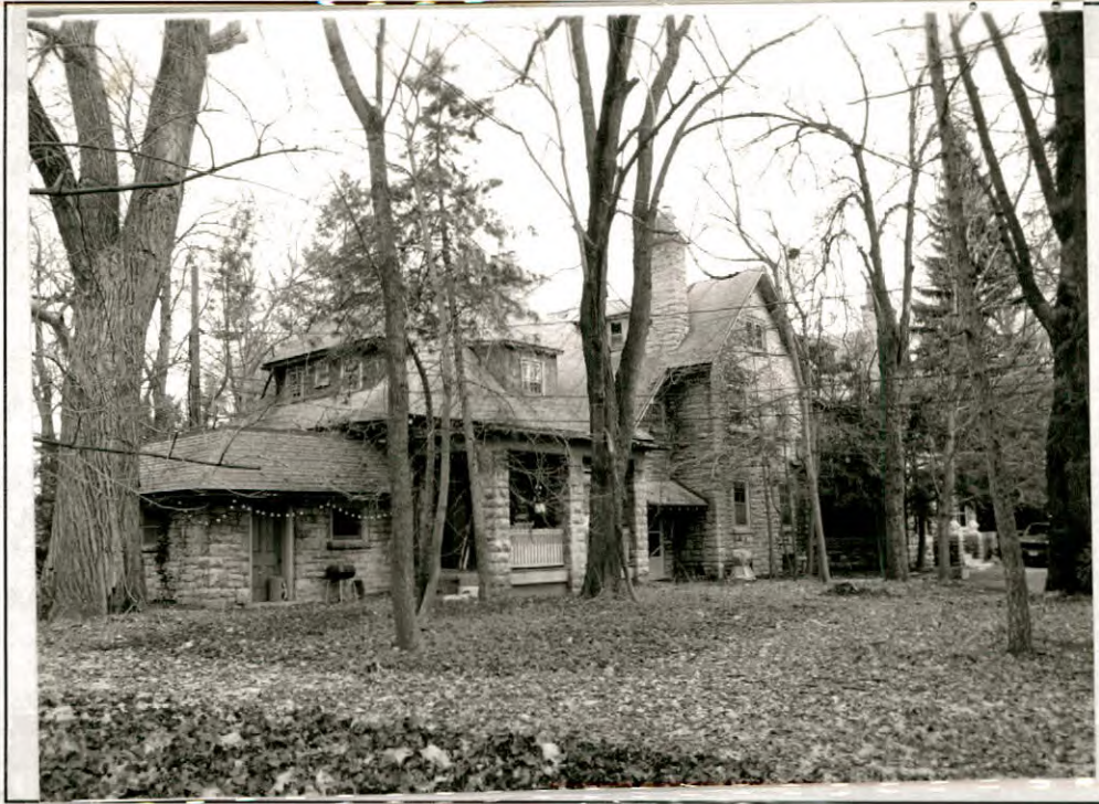
50 Getzville Road. West and south elevations.
