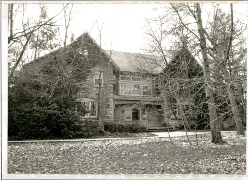
50 Getzville Road. North elevation.
