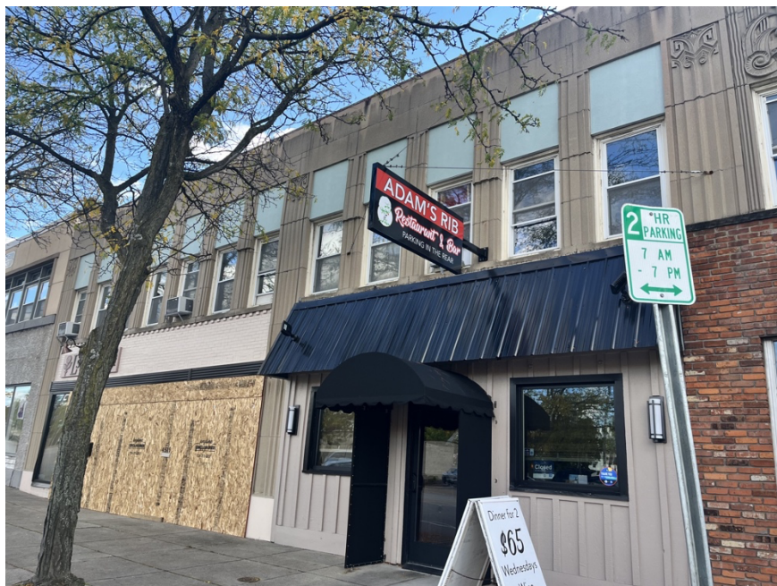
Figure 16. Primary (north) Façade, Hallie Wright
