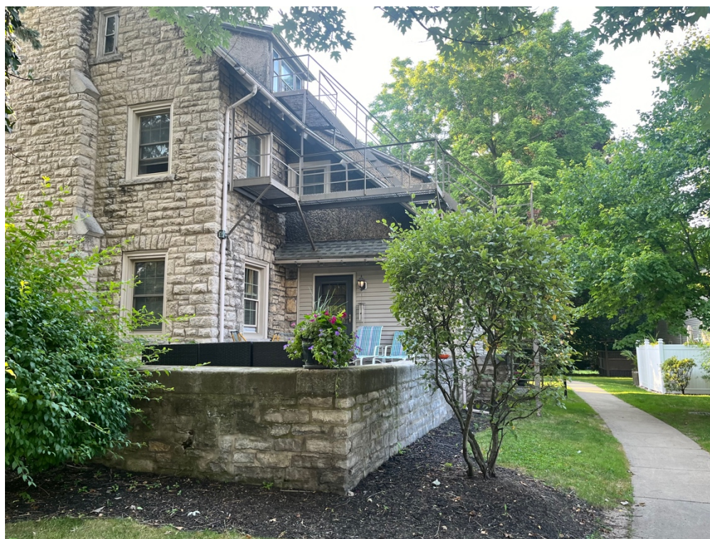
Figure 2. Southeast Elevation, Including Porch
