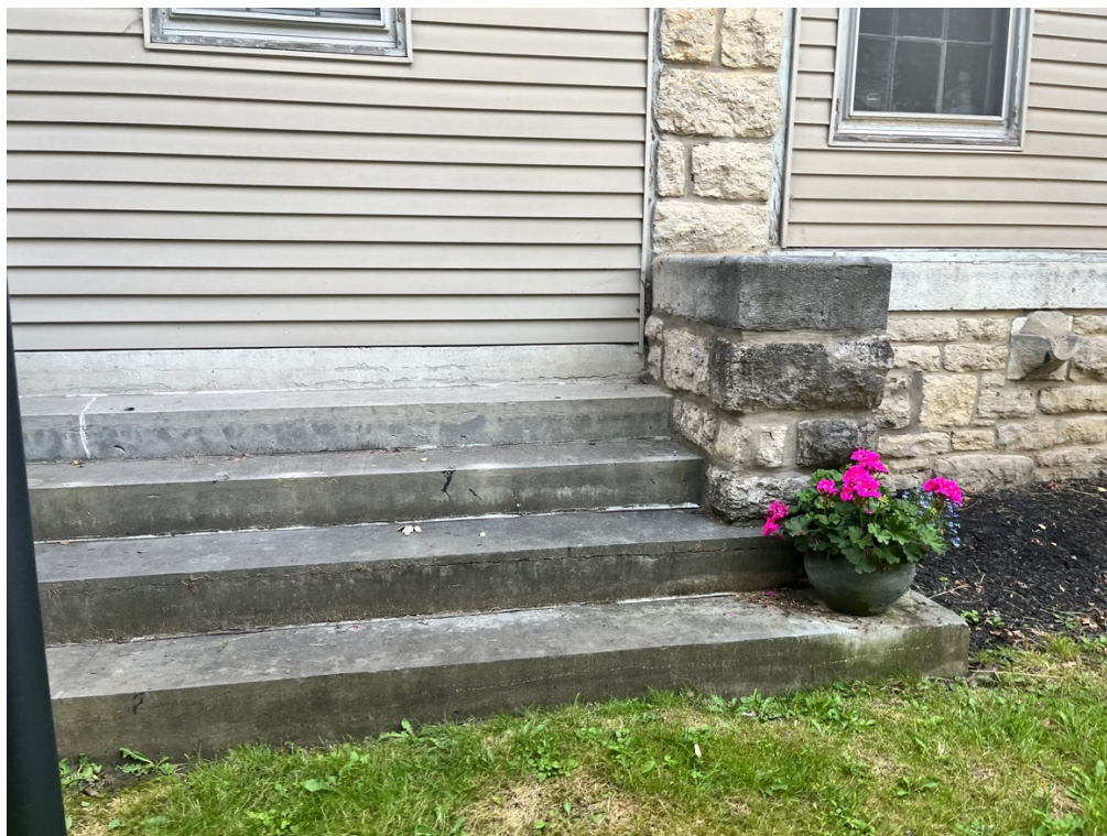
Figure 3. Southeast Elevation, Including Steps and Vinyl Siding
