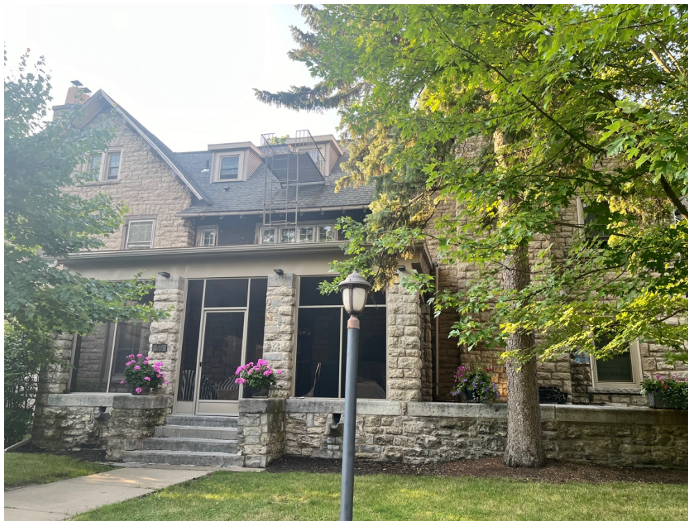
Figure 1. Primary (South) Façade
