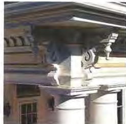
The intricate cornice-supporting brackets for the overhanging roof are also original features.
