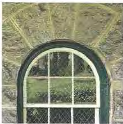
These diamond-patterned window lights are original, and characteristic of the Victorian era.
