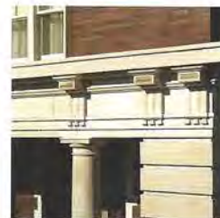
Hand-crafted columns and trim in the Italian Renaissance Revival style highlight the main entrance.
