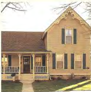
THE ROMEO HOUSE Romeo, Michigan Built in 1871 A & G Properties, Inc., Contractor. Grand Manor Shangle® in Brownstone, 32 Squares. Listed with the Romeo Historic Society, 1994.
