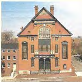
ORCHARD STREET CHURCH Headquarters for the Baltimore Urban League Baltimore, Maryland Built in 1883 Kelly, Clayton & Mojzisek, Architects, Project Architect. Struever Bros., Eccles & Rotuse, Inc., General Contractor. Grand Manor Shangle® in Stately Black®, 100 Squares. Listed on the National Register of Historic Places, 1975.
