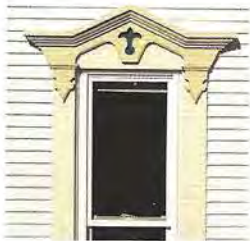
The cornice window frames and their ornate trim are representative of the Greek Revival style of architecture and are original to the house.
