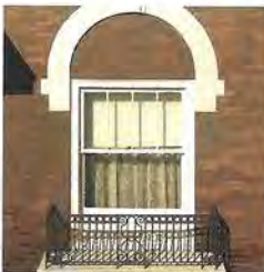
The ground-level front windows feature stone arches and extended platforms surrounded by wrought iron grillwork.
