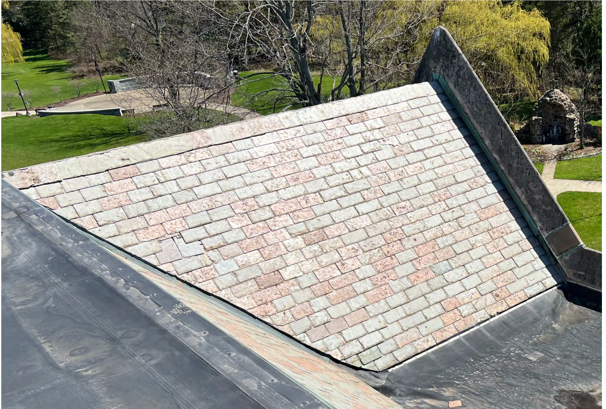
Photo of existing slate taken in May of 2022.
