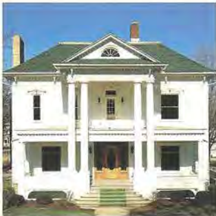
THE MONTPELIER WHITE HOUSE Montpelier, Ohio Built in 1877 Gray's Construction Company, Contractor. Carriage House Shangle™ in Sherwood Forest, 21 Squares. Application submitted, National Register of Historic Places.
