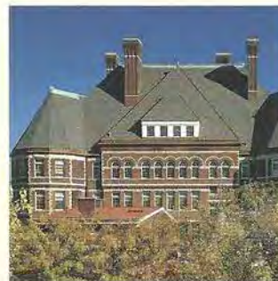
THE FAIRVIEW GERMAN BILINGUAL SCHOOL Cincinnati, Ohio Built in 1888 SFA Architects, Project Architect. Imbus Roofing, Roofing Contractor. Grand Manor Shangle® in Stonegate Gray, 230 Squares.
