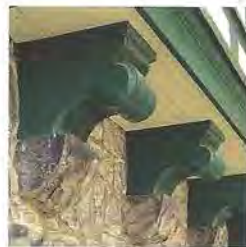
Massive hand-carved brackets extend from the heavy masonry base to support the upper stories.
