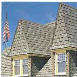
A pair of dormer windows adorns the roof on the south side of the firehouse. Deteriorating wood shingles which covered the walls of these dormer windows had to be replaced.
