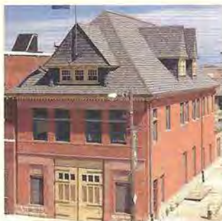
DETROIT FIRE HOUSE No. 5 Detroit, Michigan Built in 1888 Detroit Cornice and Slate, Contractor. Grand Manor Shangle® in Stonegate Gray, 65 Squares. Listed on the National Register of Historic Places.
