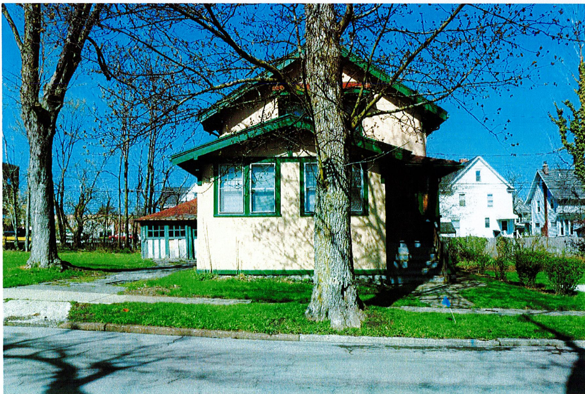
4. Direct view of east elevation, facing west ( Commonwealth 2022 ).
