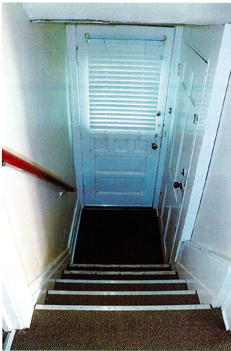
29. View of side entrance hall with basement door at right, facing north ( Commonwealth 2022 ).
