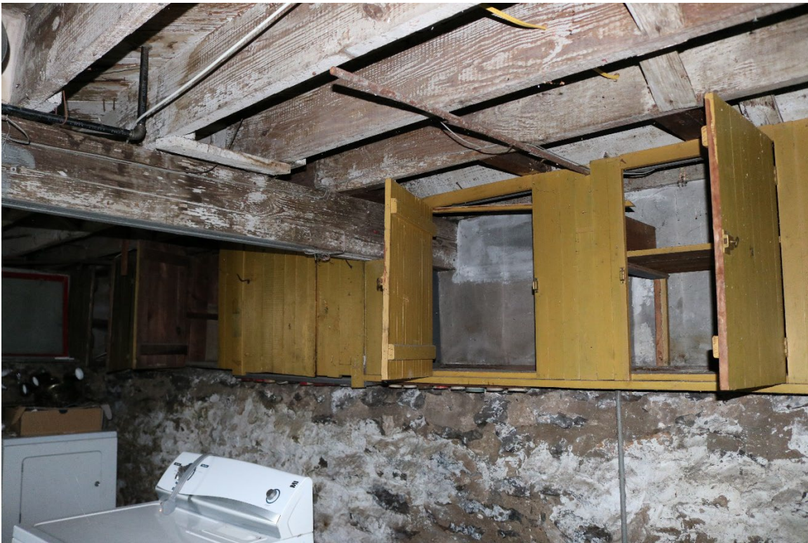
43. Detail of west basement wall, facing southwest ( Commonwealth 2022 ).
