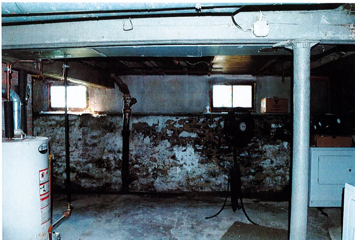
44. View of basement, facing north ( Commonwealth 2022 ).
