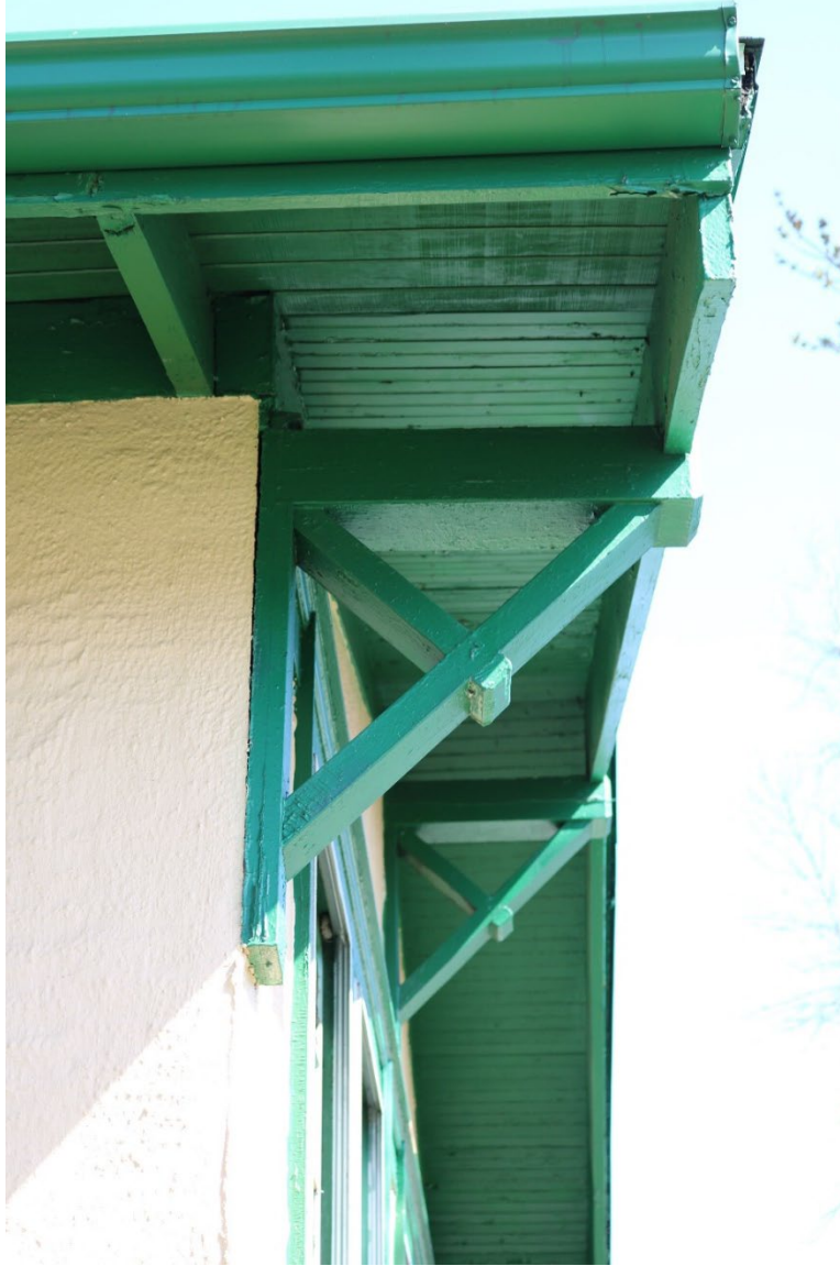
7. Detail view of brackets and eaves, facing northwest ( Commonwealth 2022 ).
