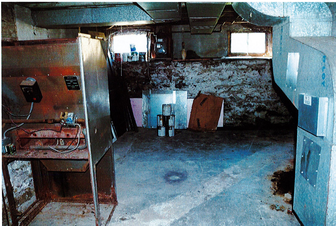
42. View of basement, facing south ( Commonwealth 2022 ).
