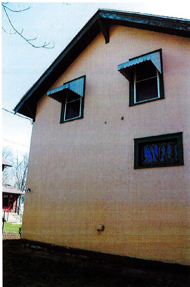
10. Oblique, partial view of the west elevation facing northeast ( Commonwealth 2022 ).
