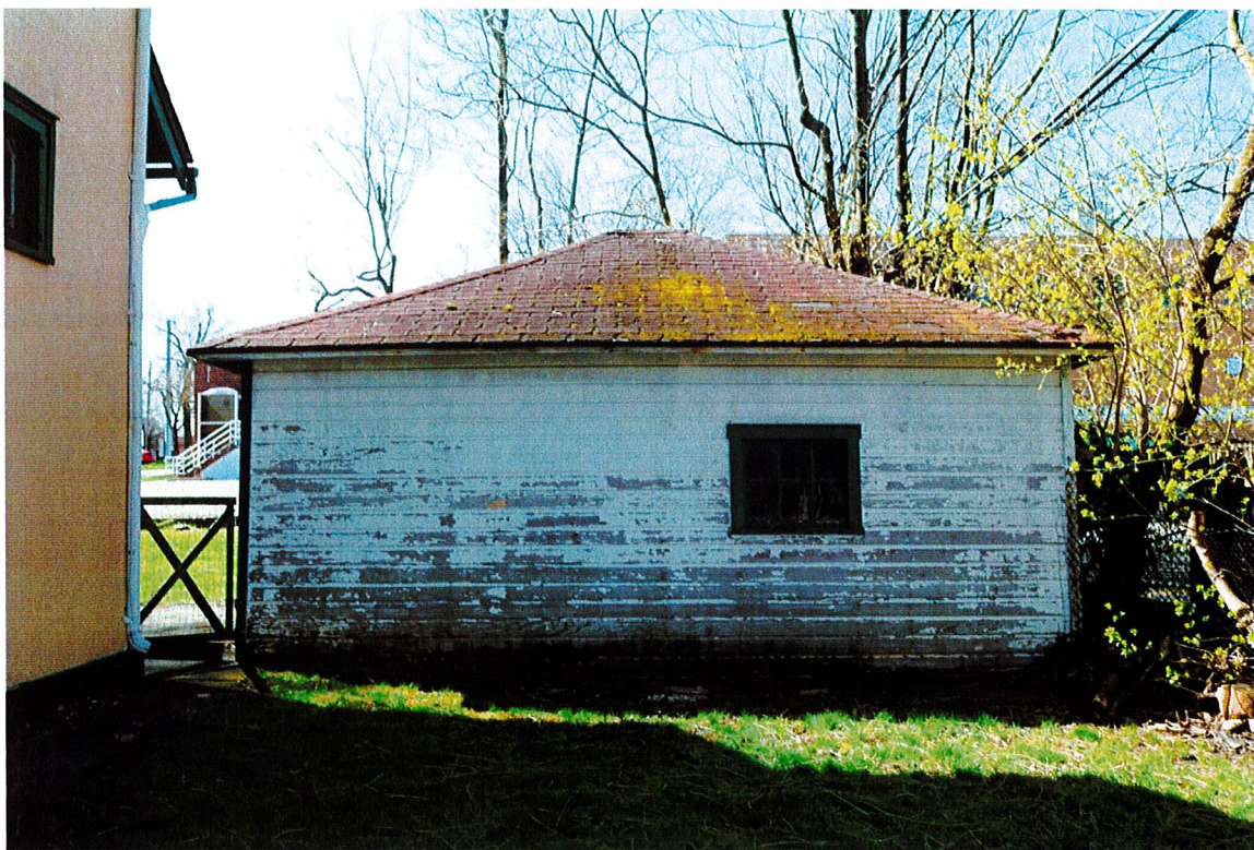
11. View of backyard and north elevation of the garage, facing south ( Commonwealth 2022 ).
