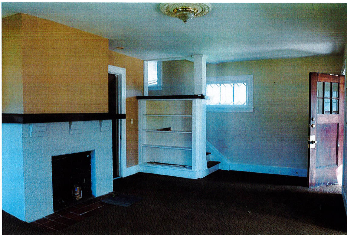
18. View of living room looking toward built-in shelves and stairs, facing northwest (Commonwealth 2022).
