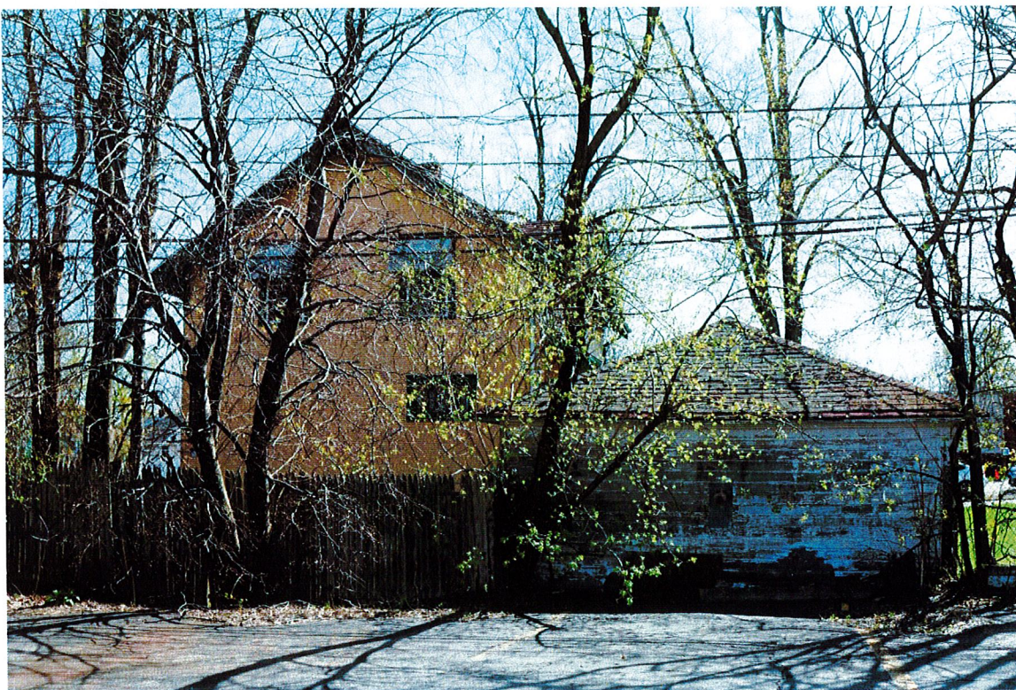
9. Direct view of west elevations of the house and garage, facing southeast ( Commonwealth 2022 ).
