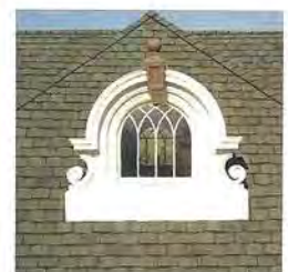
Ornate dormer windows extend from the third story on each side of the house.
