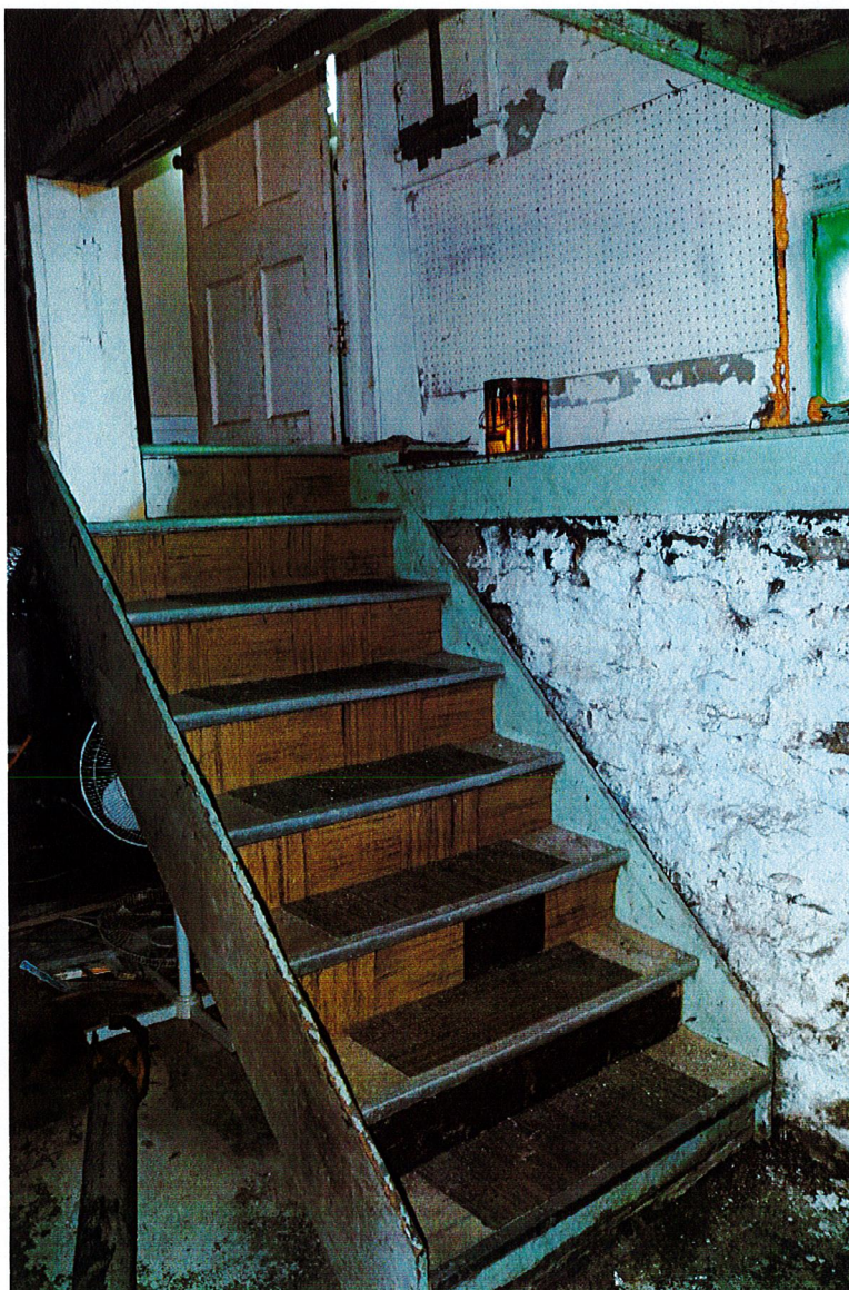
41. Detail of basement stairs, facing northwest ( Commonwealth 2022 ).
