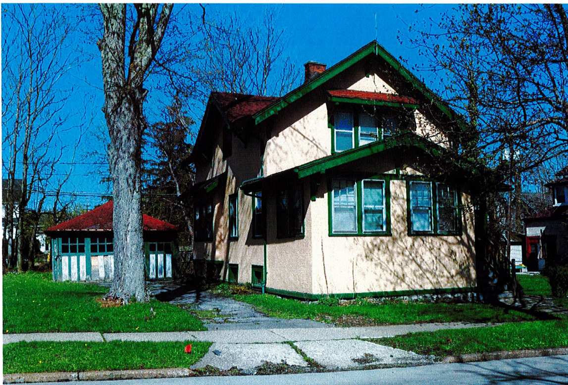
3. Oblique view of south and east elevations, facing west-northwest ( Commonwealth 2022 ).
