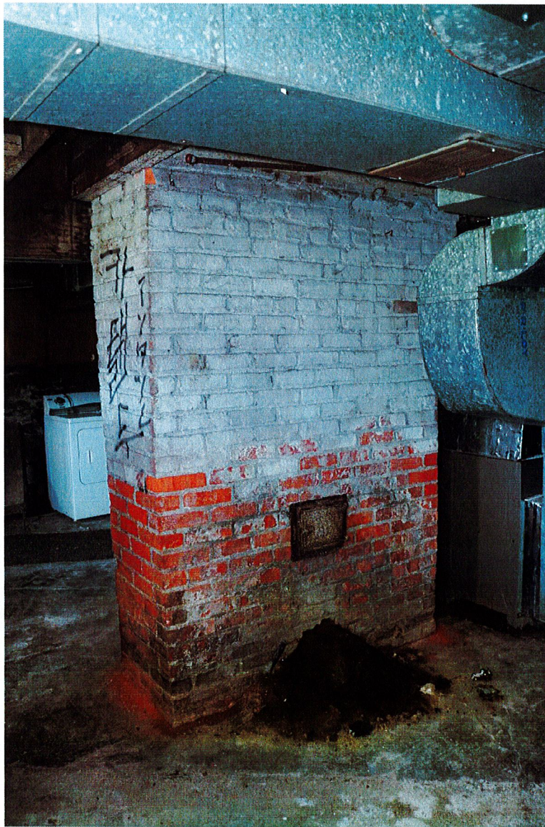
45. View of basement, facing west-northwest ( Commonwealth 2022 ).
