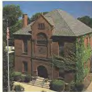
NORTH KINGSTOWN TOWN HALL North Kingstown, Rhode Island Built in 1890 Pezzucio Construction Company, Contractor. Grand Manor Shangle® in Stonegate Gray, 50 Squares. Listed on the National Register of Historic Places.
