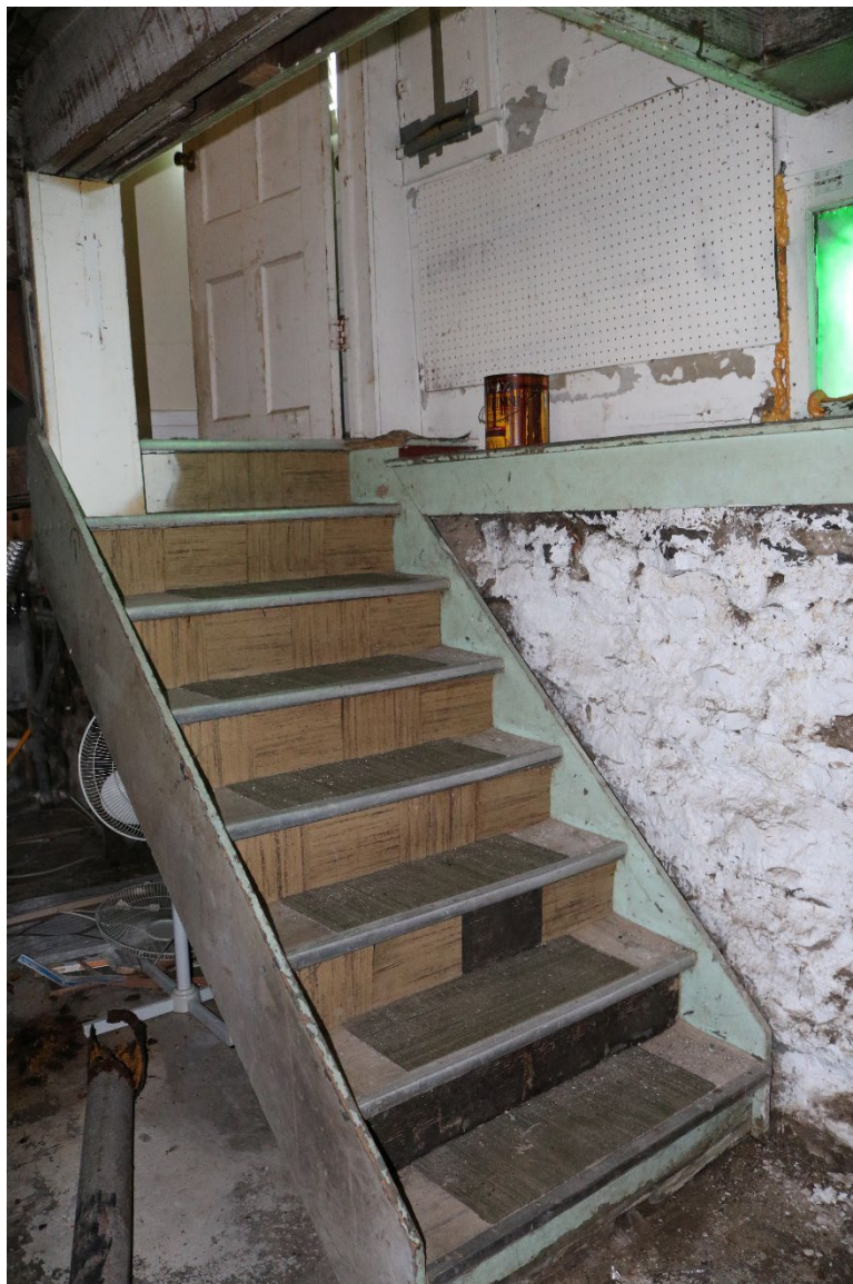
41. Detail of basement stairs, facing northwest ( Commonwealth 2022 ).
