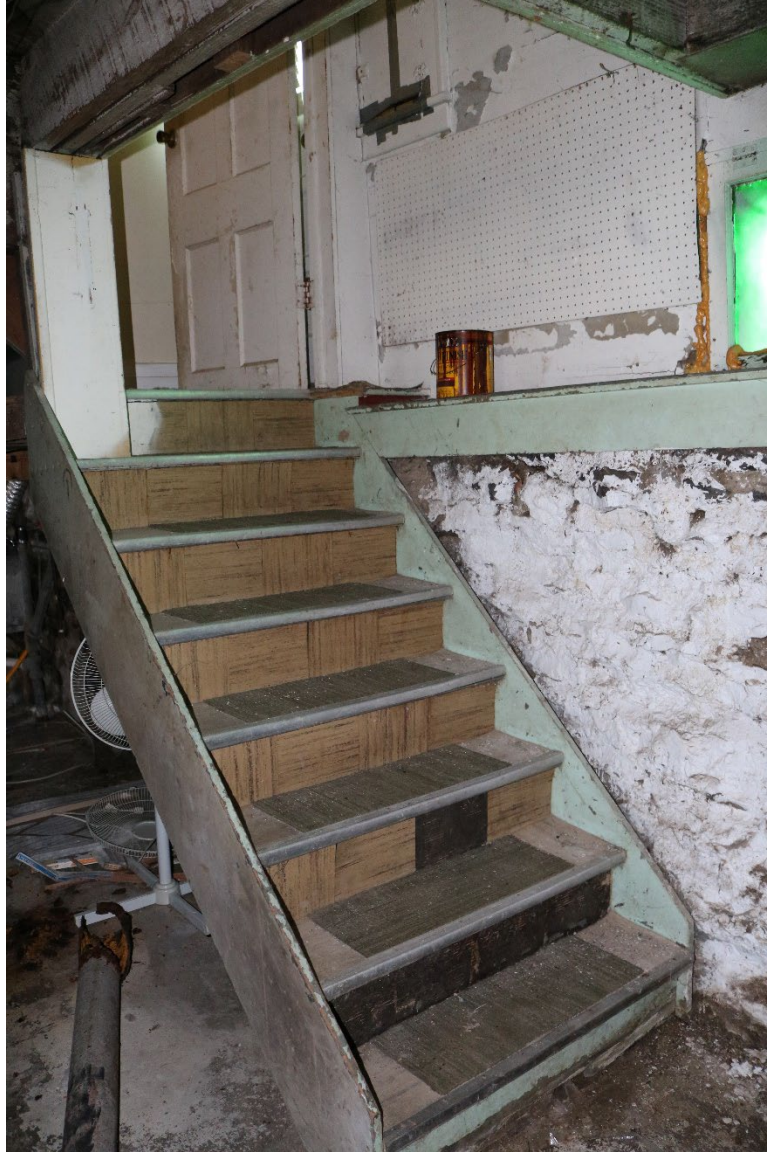
41. Detail of basement stairs, facing northwest ( Commonwealth 2022).
