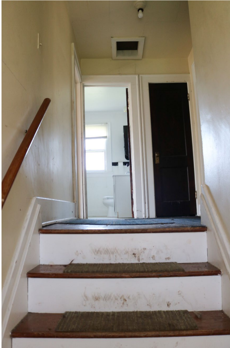
31. View of 2 nd floor hall from staircase landing with bathroom at left and closet at right, facing south ( Commonwealth 2022).
