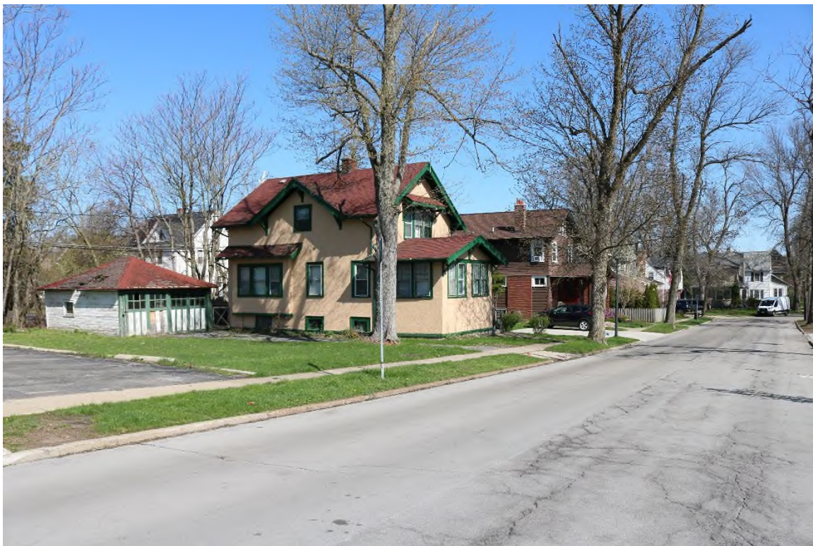
1. Setting view of 22 Chateau Terrace, facing northwest ( Commonwealth 2022 ).
