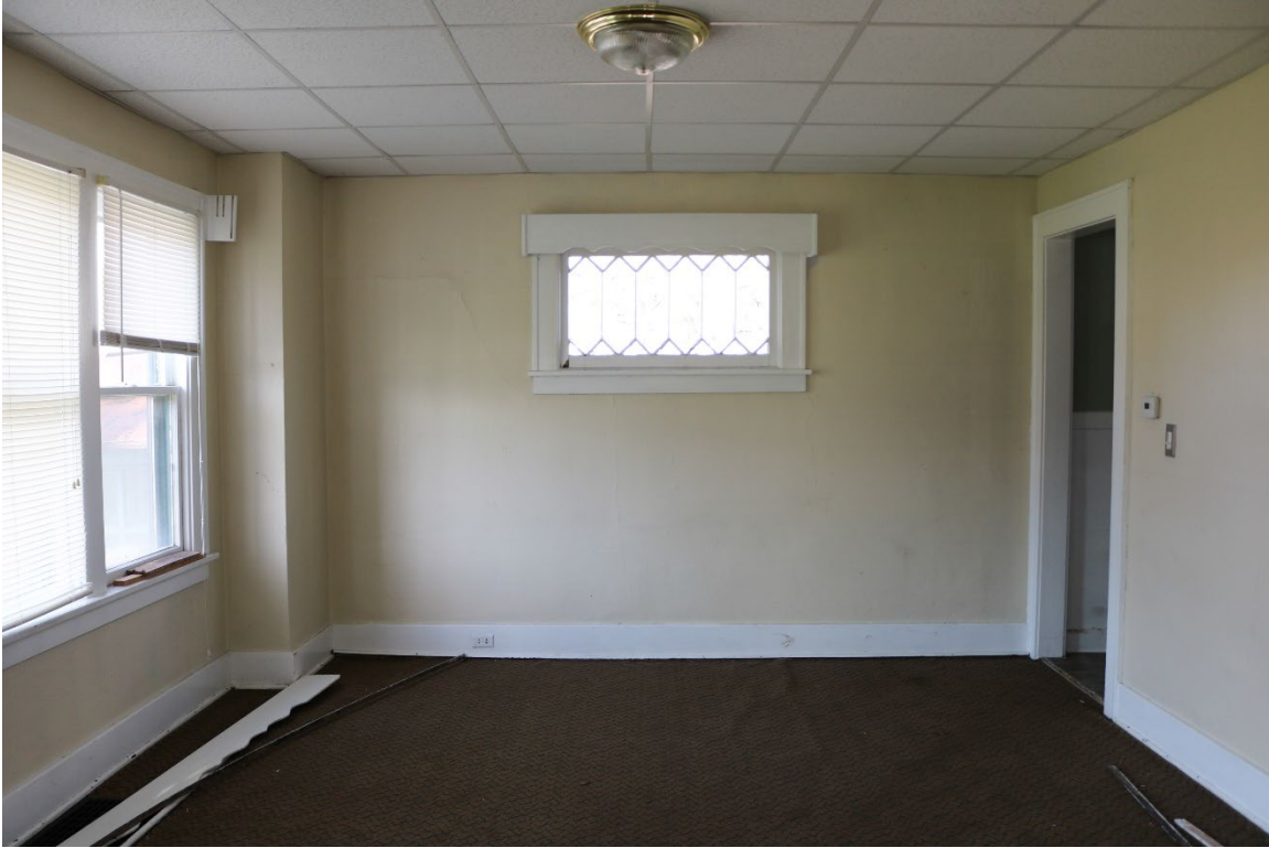
22. View of dining room, facing west ( Commonwealth 2022 ).
