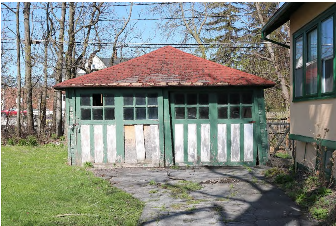
13. Direct view of north elevation of garage, facing west ( Commonwealth 2022 ).
