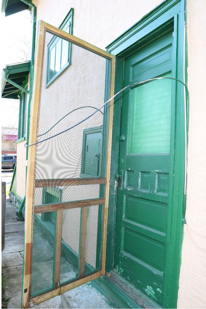
8. Detail view of entrance on north elevation, facing southeast ( Commonwealth 2022 ).
