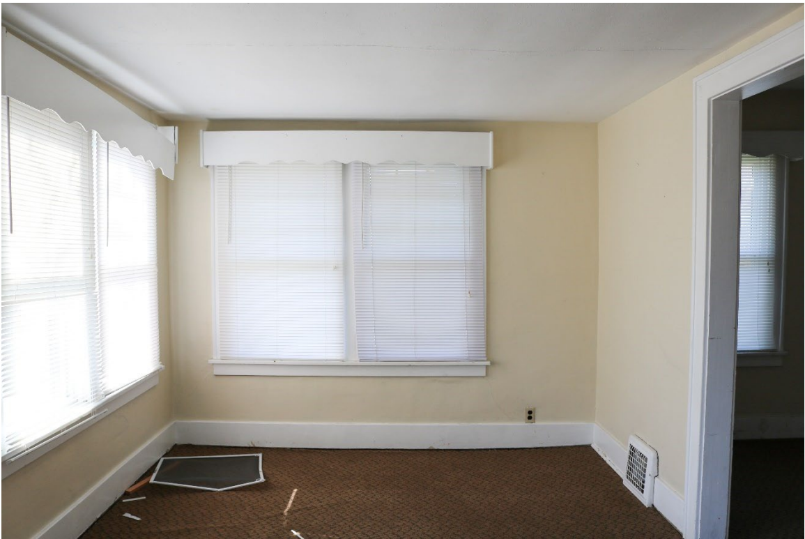
21. View of first floor sunroom, facing south ( Commonwealth 2022 ).
