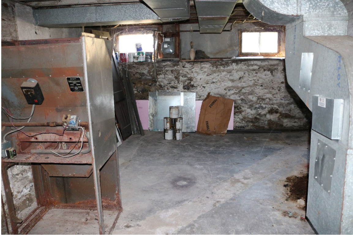
42. View of basement, facing south ( Commonwealth 2022 ).
