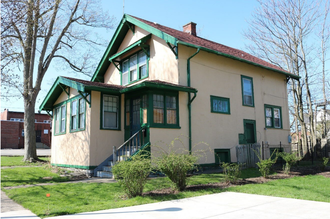
5. Oblique view of east and north elevations, facing southwest ( Commonwealth 2022 ).
