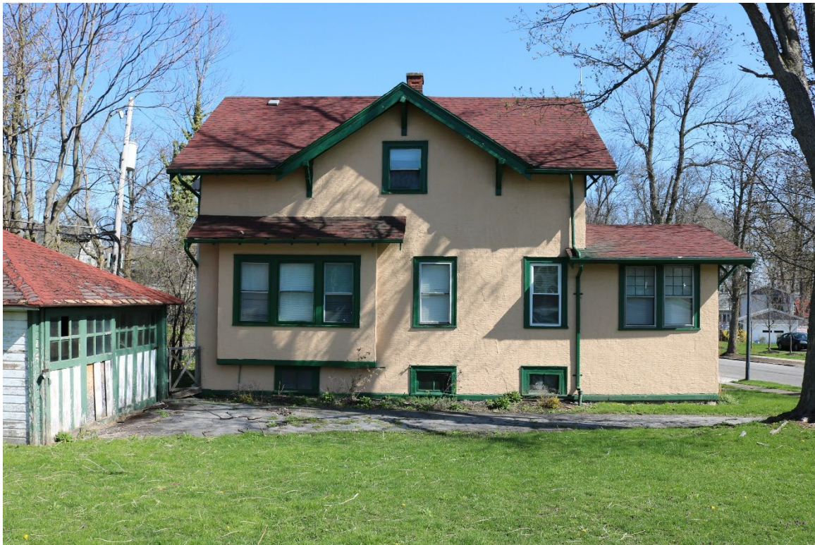
12. Direct view of south elevation, facing north ( Commonwealth 2022 ).
