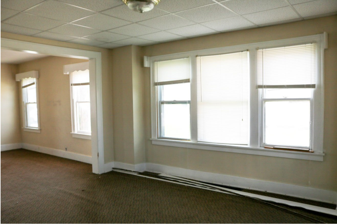
24. View of east wall of first floor from dining room, facing southeast
