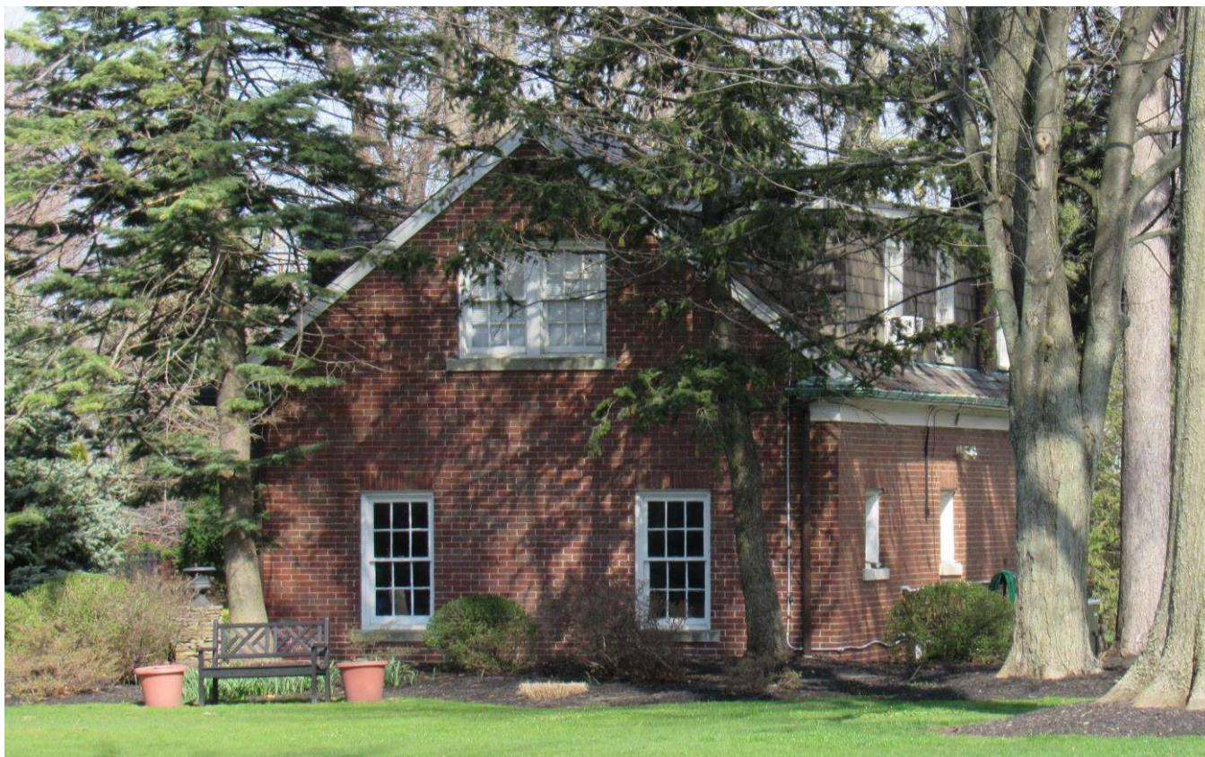
NY_Erie County_Town of Amherst_725 LeBrun Road_Detached Garage
